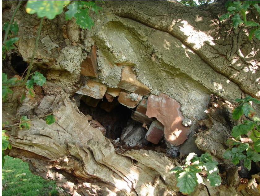
The large cavity partly filled by concrete and bricks in the main trunk ( Target Note 5 ).
