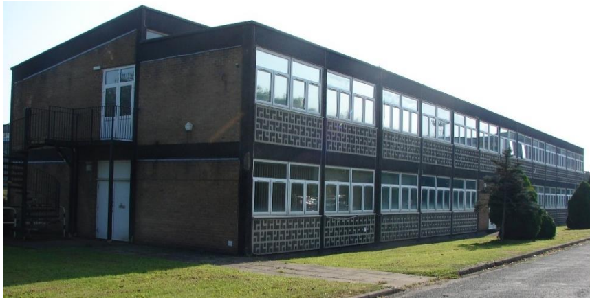
The northern and western elevations.
