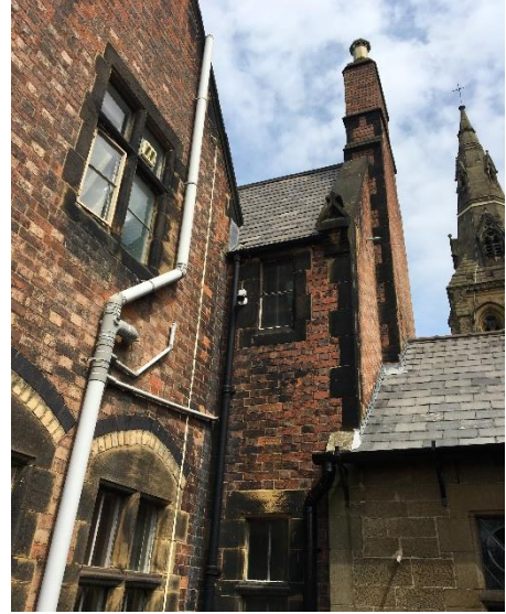
Stone mullions on adjacent windows
