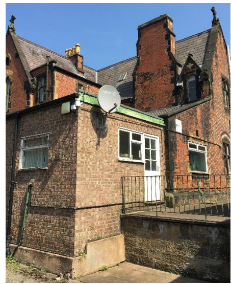
East elevation of the scullery extension
