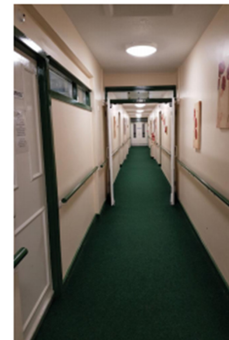
6 Existing Circulation Space
