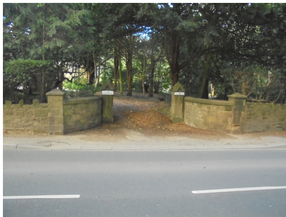
Existing Main Access
