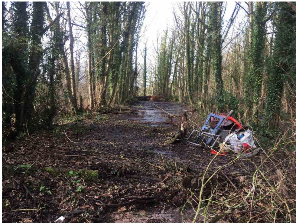
Photo 2. Area on the Southern boundary showing concrete pad of hospital building with tree line either side of it
