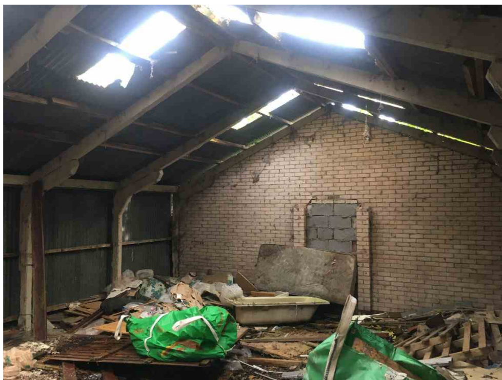
Photo12. Building B2 internal with large amount of light ingress and steel walls and roof
