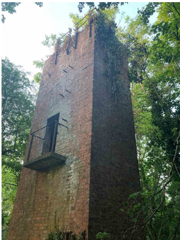
Photo 7. Building B1 the water tower. Southern and eastern aspects. Note access to first floor
