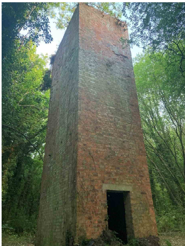
Photo 8 Building B1 the water tower. Western and northern aspects. Note access to ground floor
