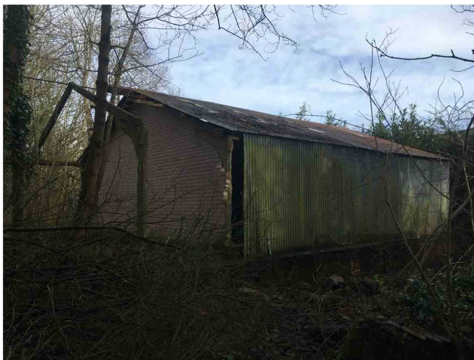
Photo 11. Building B2, steel sheet walls and roof
