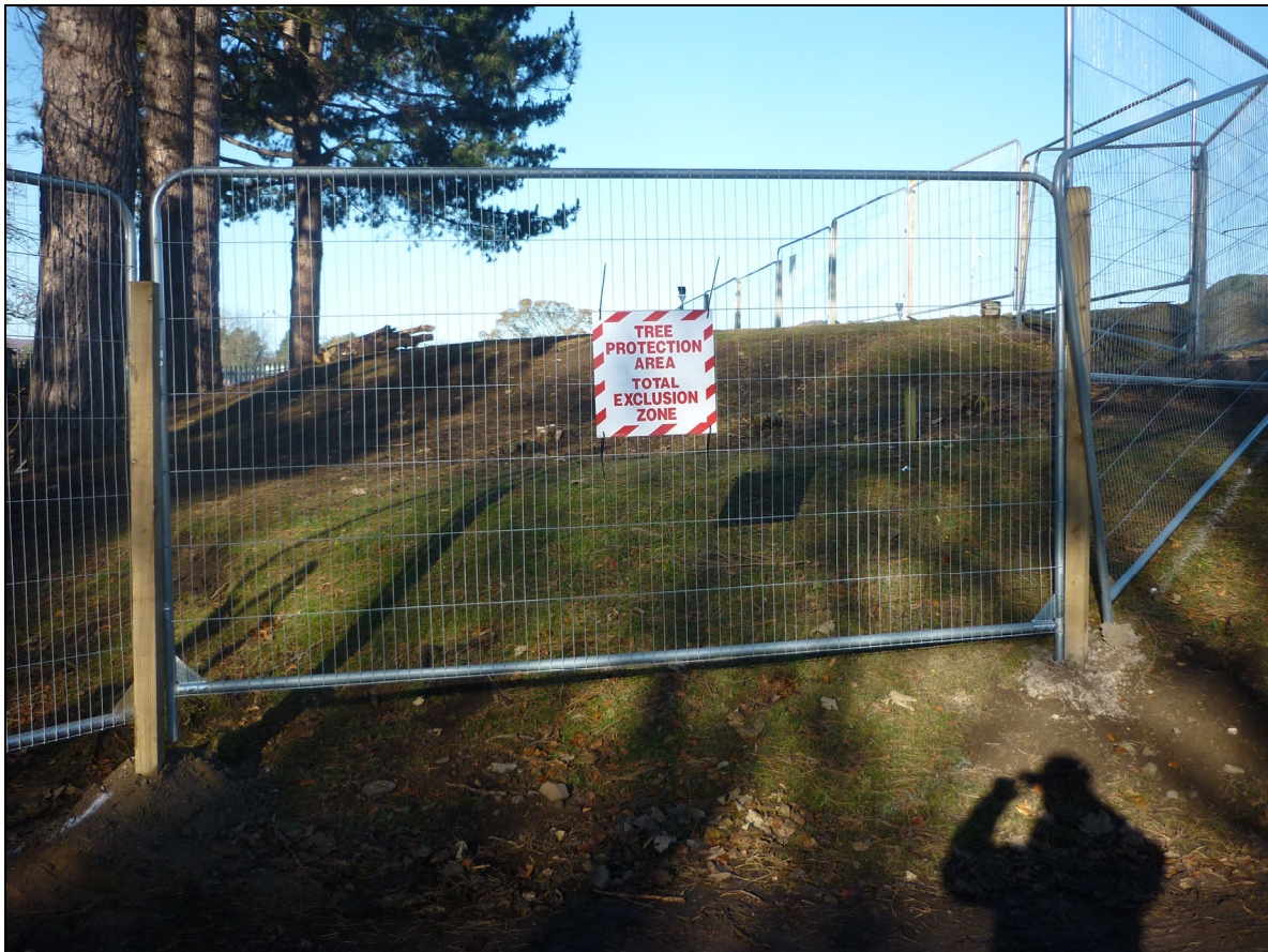
Tree Protective Fencing Specification
