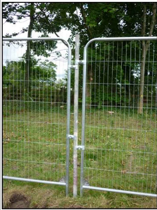
Tree Protective Fencing Specification
