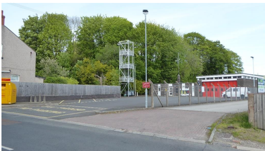
Figure 4.6. Land west of site
