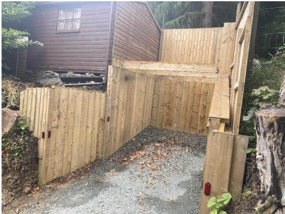
Plate 1: Car parking space at Pistyll Y Garth
