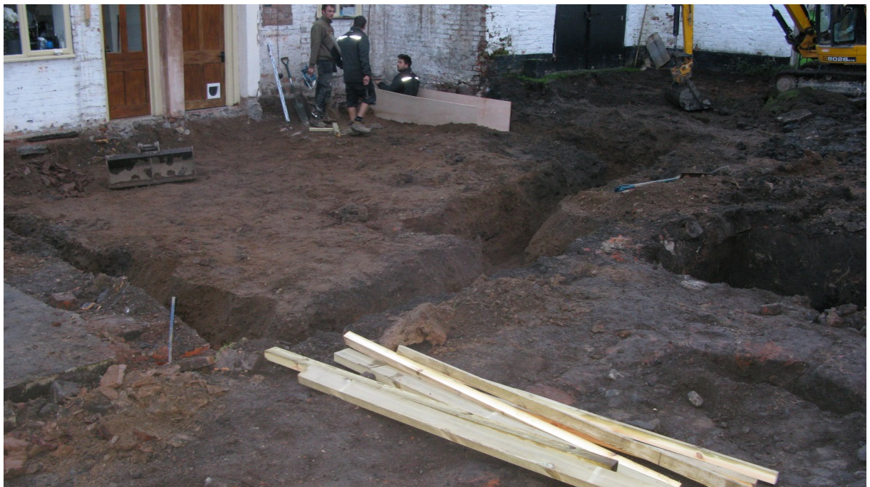
Trenches 1–5 from the north-west. Alan Wilmshurst
