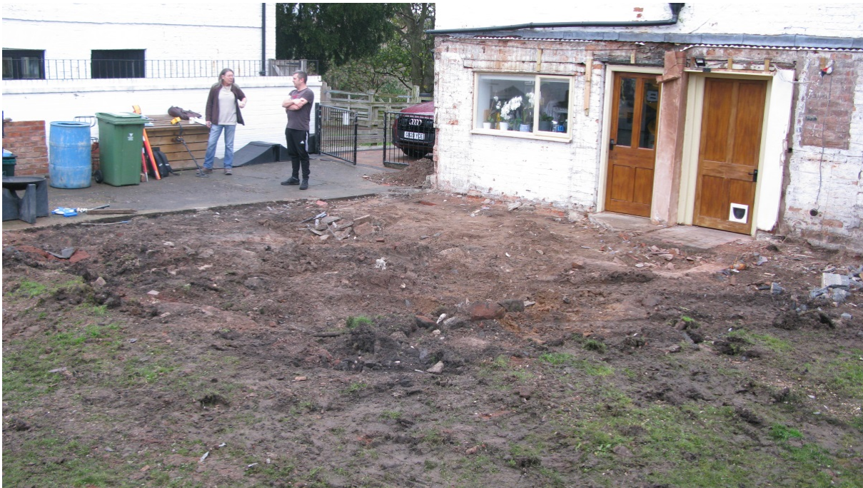
The site prior to excavation from the south-west. Alan Wilmshurst
