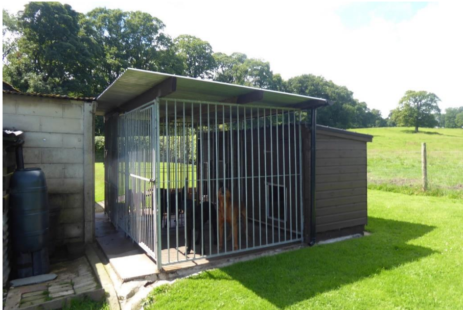
Figure 4.7. Kennels from east
