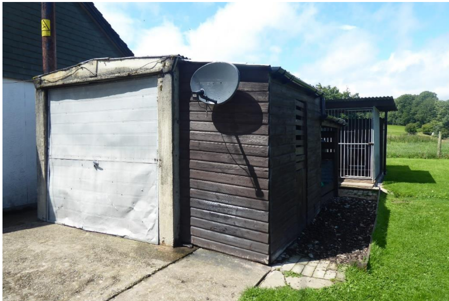
Figure 4.6. Garage from south
