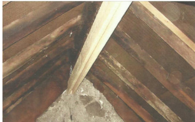
Figure 20: Crevice box in loft void.
