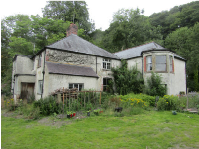
Photo 4: East elevation of the derelict building.
