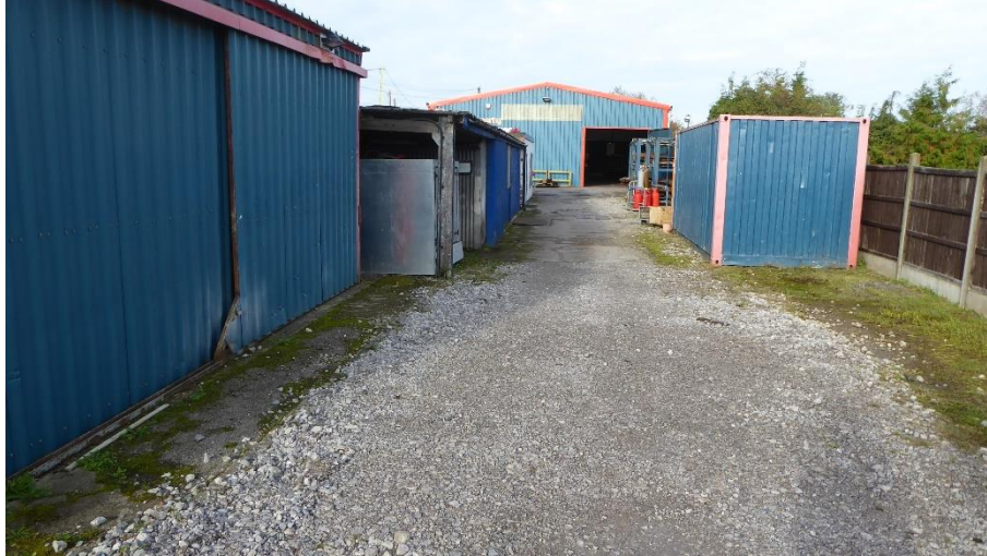
Figure 4.2. Hardstanding along northern edge of site
