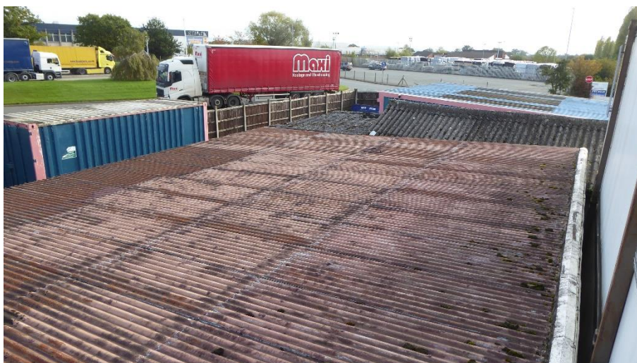
Figure 4.7. Flat roofs with no cavity
