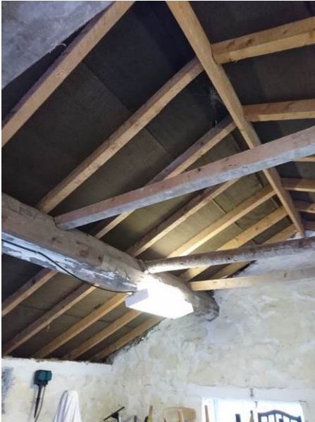
Typical view of roof.
