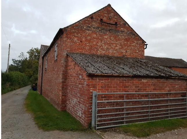
South facing gable of west wing
