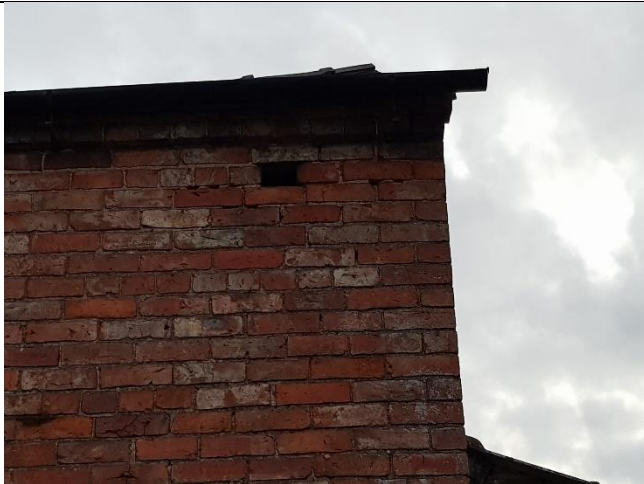
Aeration brick in use as an entry point into the loft
