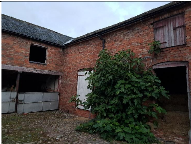
Part of the hay loft at the west end of the north wing of the barn will be included within the conversion
