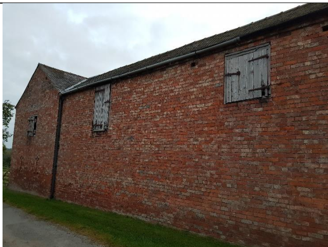
North facing elevation of the barn
