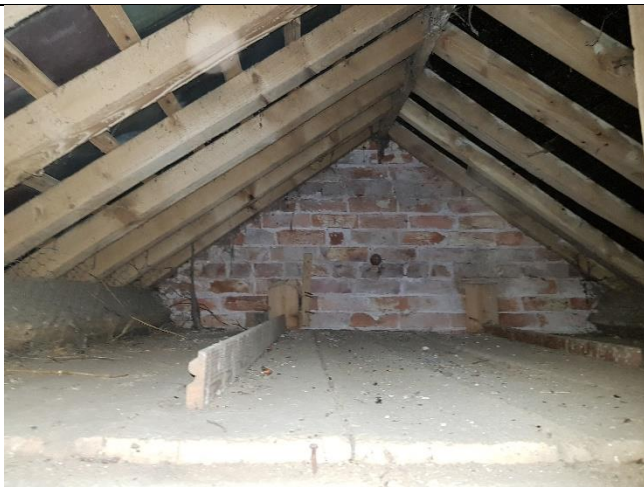
Internal loft space above west wing
