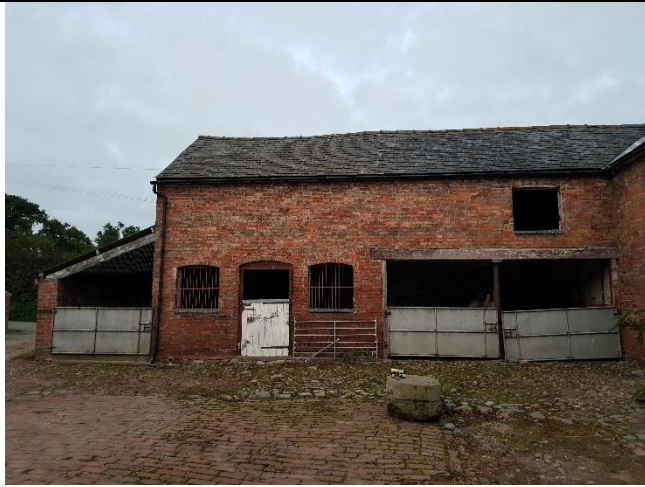
West wing of the barn to be converted
