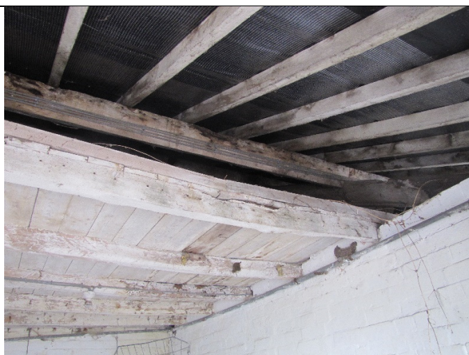
STABLE BLOCK INTERNAL SHOWING SHALLOW LOFT ABOVE PART-CEILING
