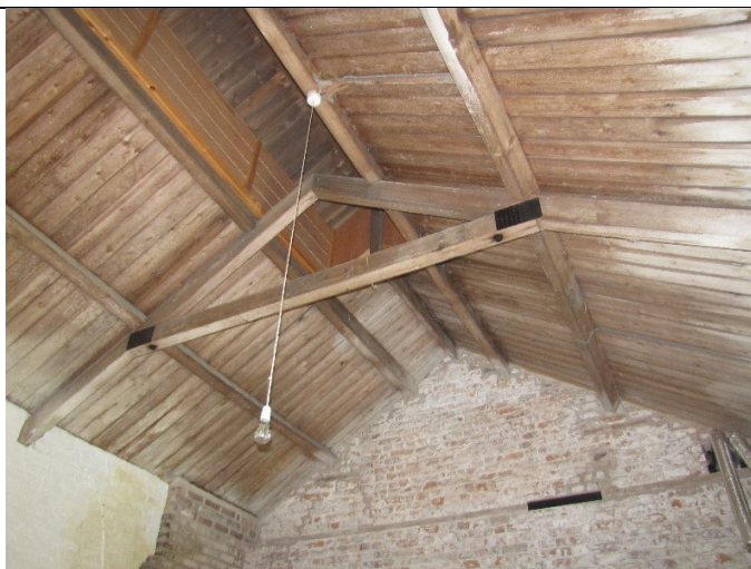
BUILDING 2 INTERNAL AT SOUTHERN END
