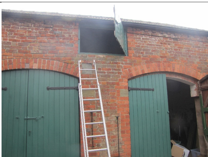
ACCESS TO LOFT IN BUILDING 3
