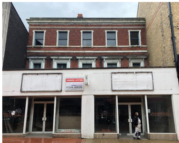
Fig I – view of front elevation of property
