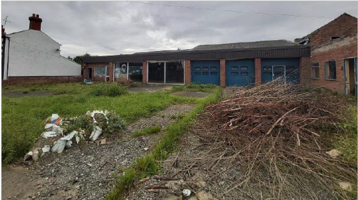
Figure 3 – The site in September 2020
