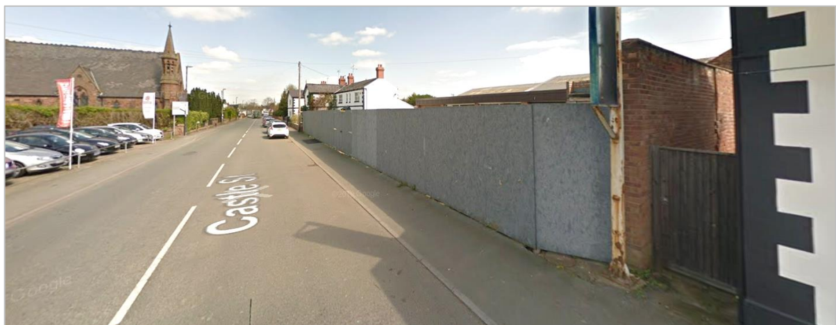
Figure 12 – Site is currently enclosed with metal fencing to the detriment of the conservation area
