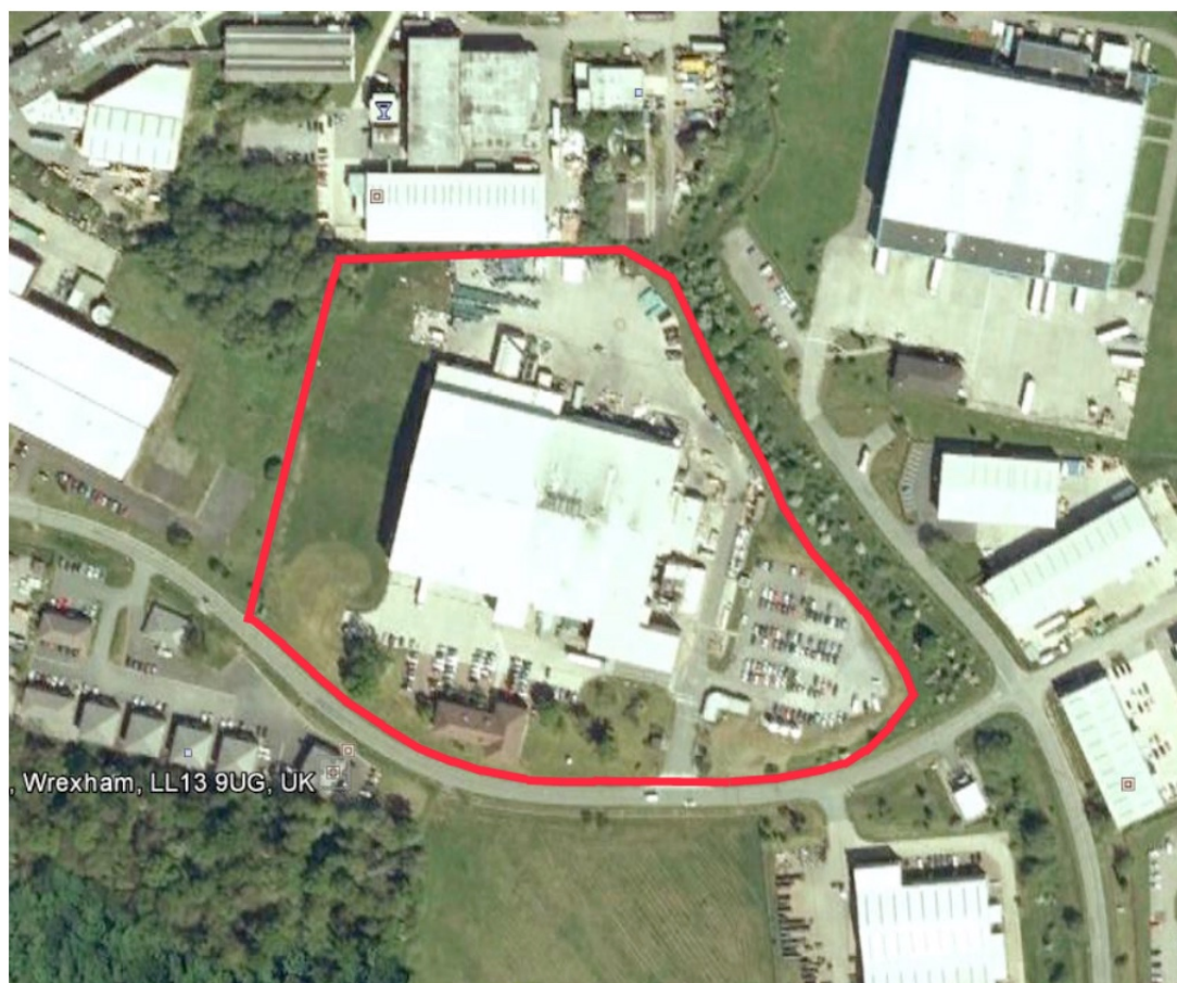
(Figure 1 – Aerial photograph of the Rowan Foods facility (Outlined in Red). Image courtesy of Google Earth, © Google)
