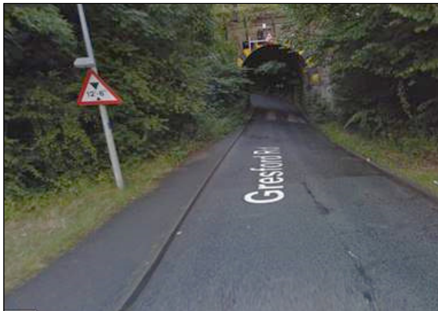
Figure 3-1: Low Bridge Preventing Access along Gresford Road
