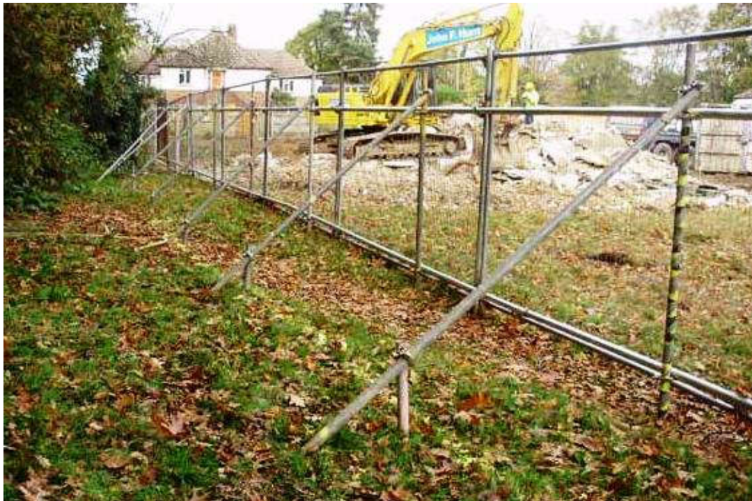
Figure 2: Photo of fencing to BS 5837:2012
