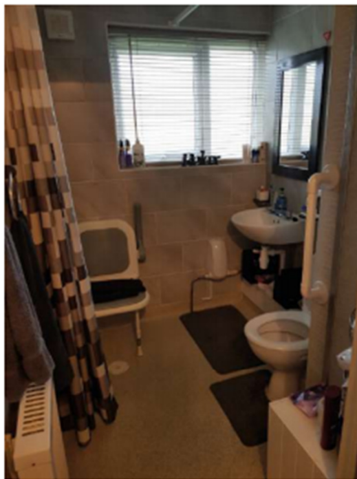
4 Existing Typical Bathroom
