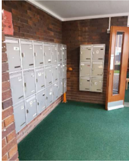
1 Existing Main Entrance
