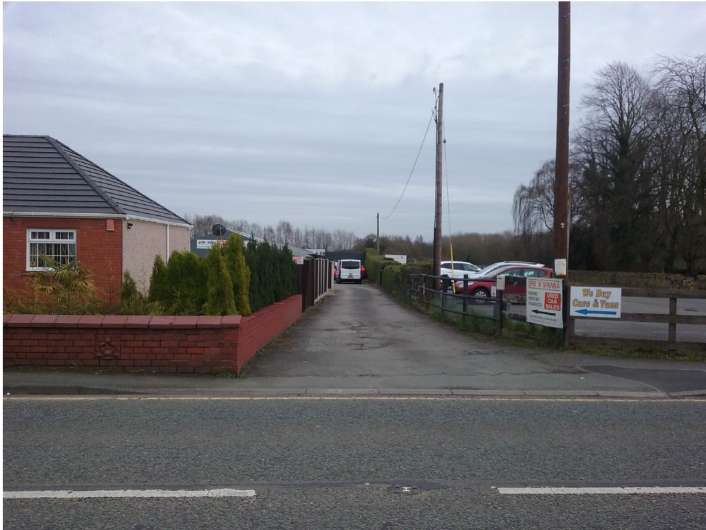
View of existing site Entrance
