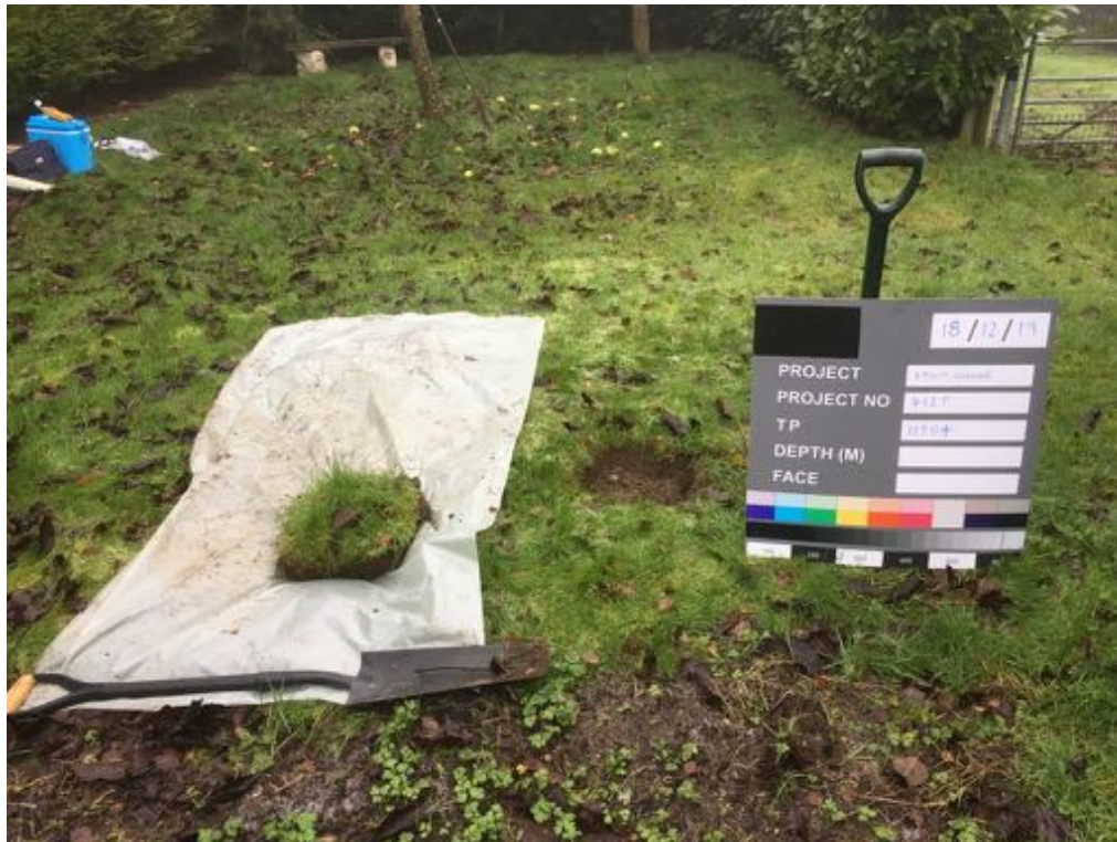
Photograph 29 Description: Hand pit HP04 Date: 18/12/2019 Location: Northern half of the orchard area
