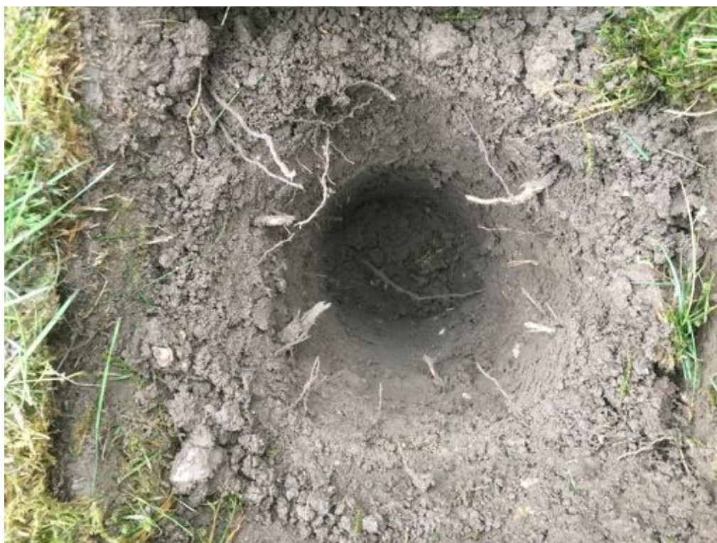
Photograph 42 Description: Hand pit HP07 Date: 18/12/2019 Location: Central part of the orchard area
