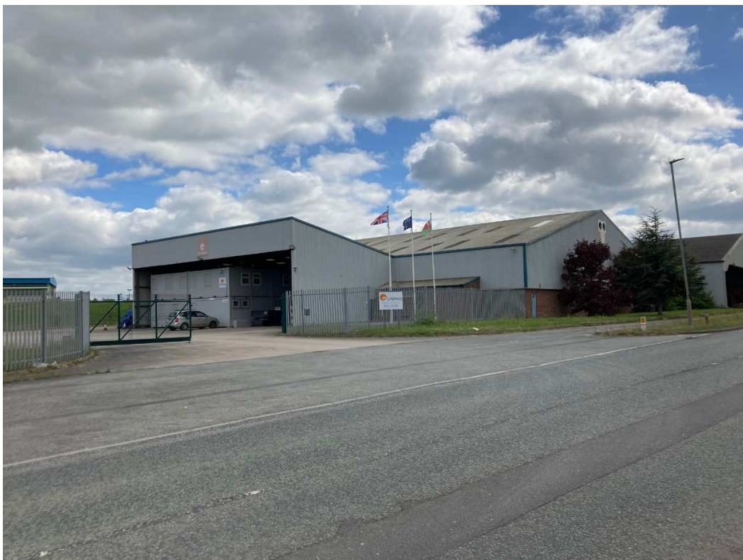
Fig 7 – Existing Unimaq building on Unit 6 – viewed from Bridge Rd North
