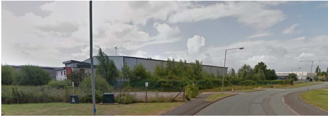
Fig 8 – Existing adjacent units to the north of Unit 6 – viewed from Bridge Road North
