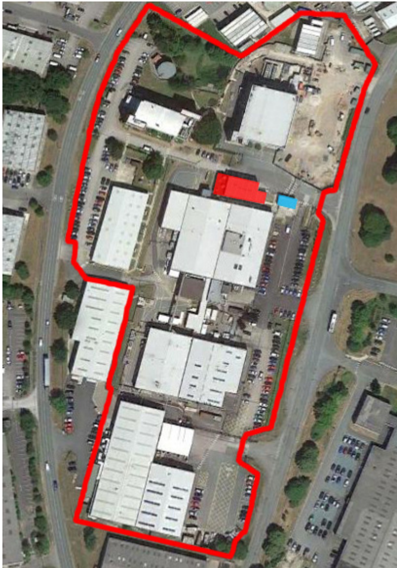
Fig 2. Aerial view of site – Existing modular building location highlighted in red, the removal of the security lodge is shown in blue.
