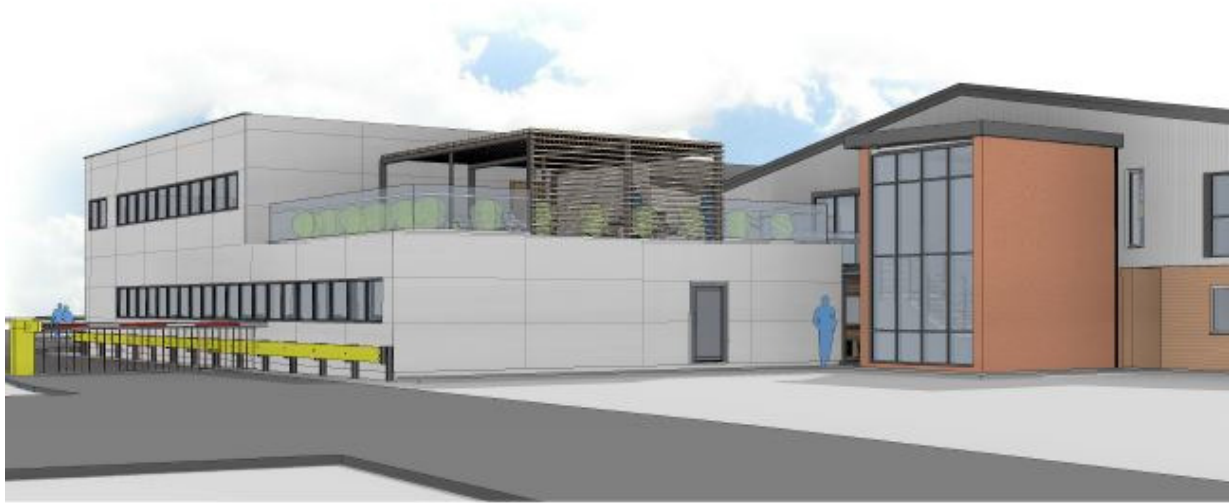
Fig 6. Existing location of Modular Office building
