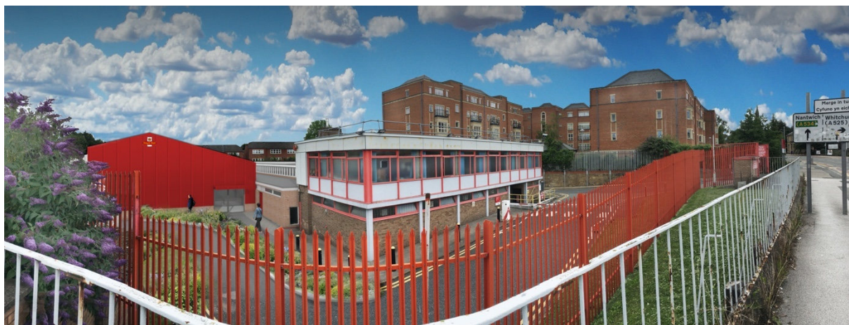
View of the new extension with planting adjacent to the customer access path.
