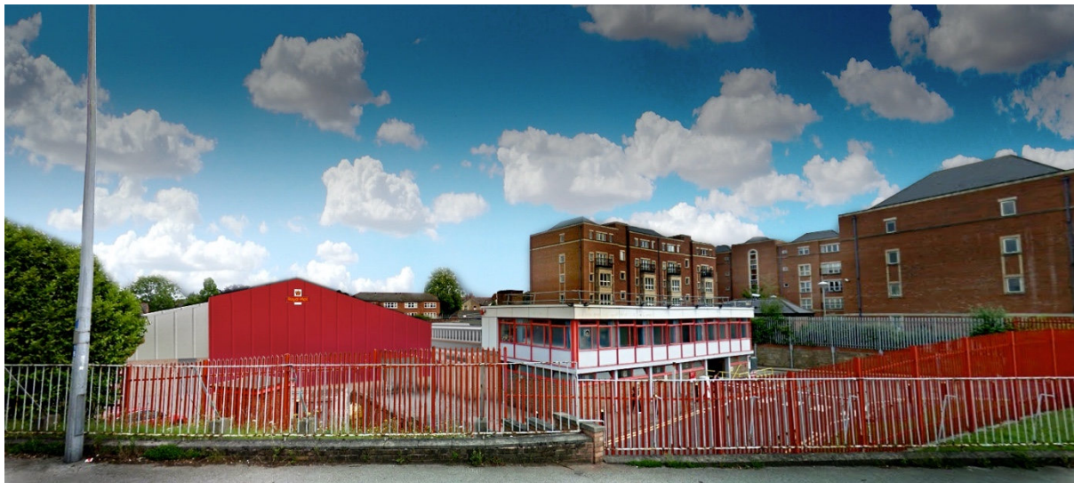
View of the new extension adjacent to the existing building as viewed from Regent Street with residential buildings to the east of the site.
