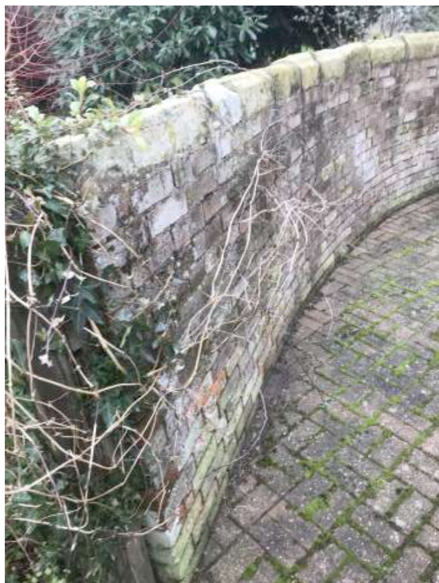
- Existing curved brick masonry wall with stone cappings.
