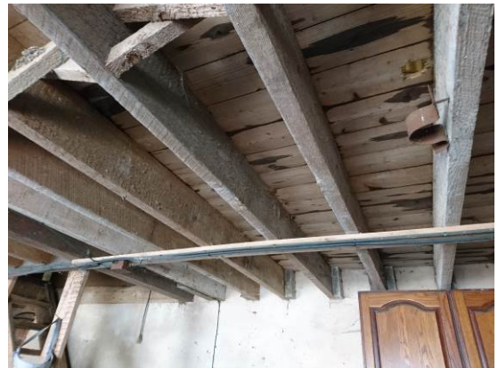
Photo 18 – General view of floor over.
