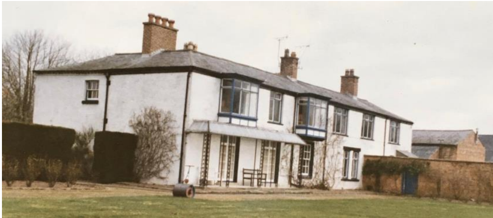
Photograph showing south elevation, circa 1970's
