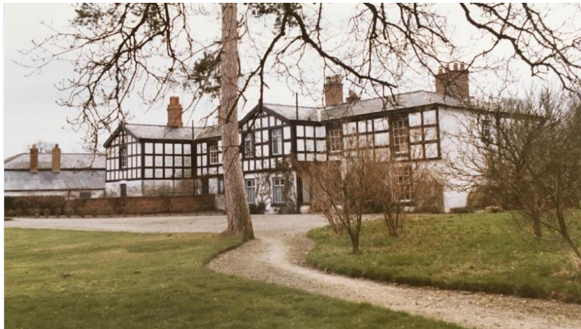
Photograph showing north elevation, circa 1970's
