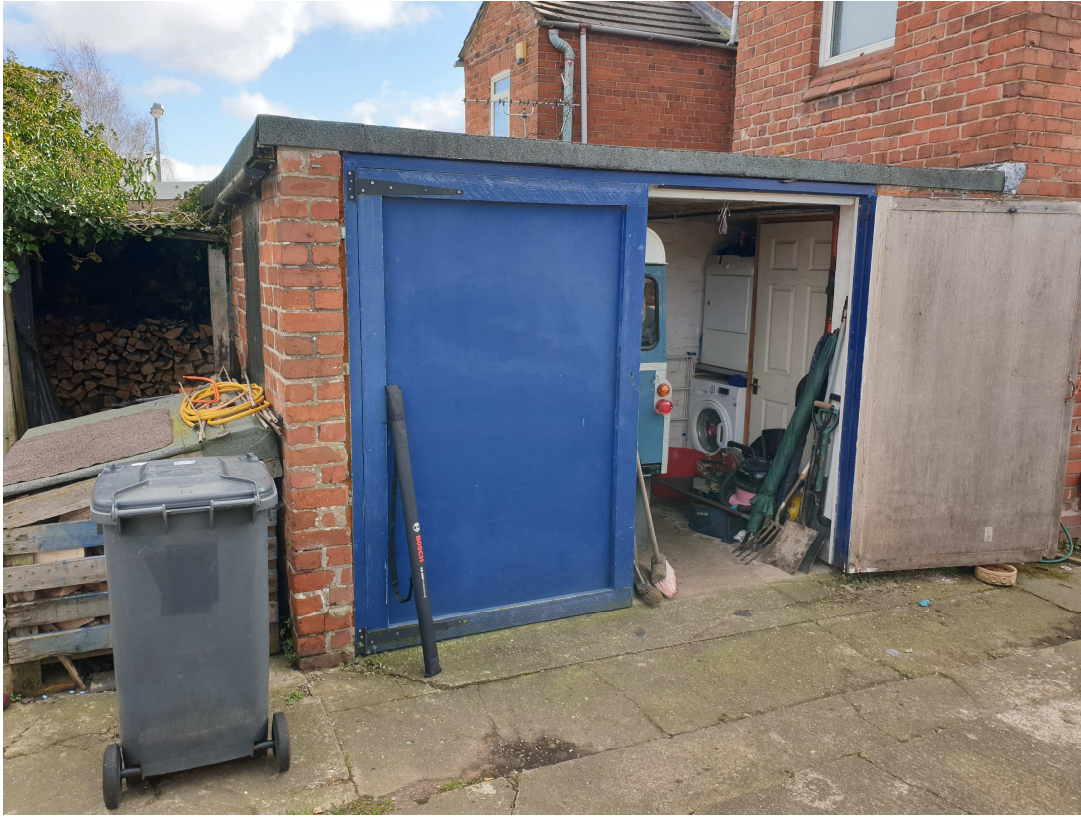
Photos of the Existing Garage
