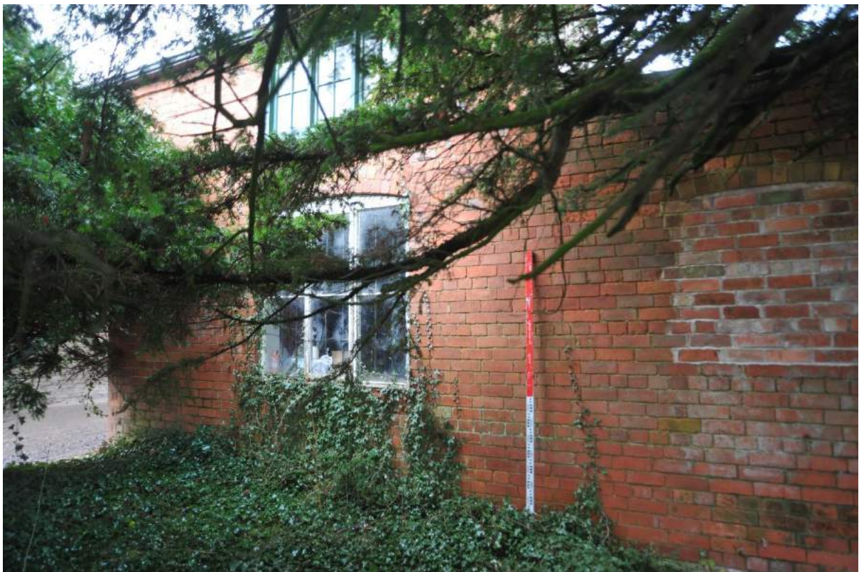
Pl.10: The northern end of the east elevation of the East Range.
