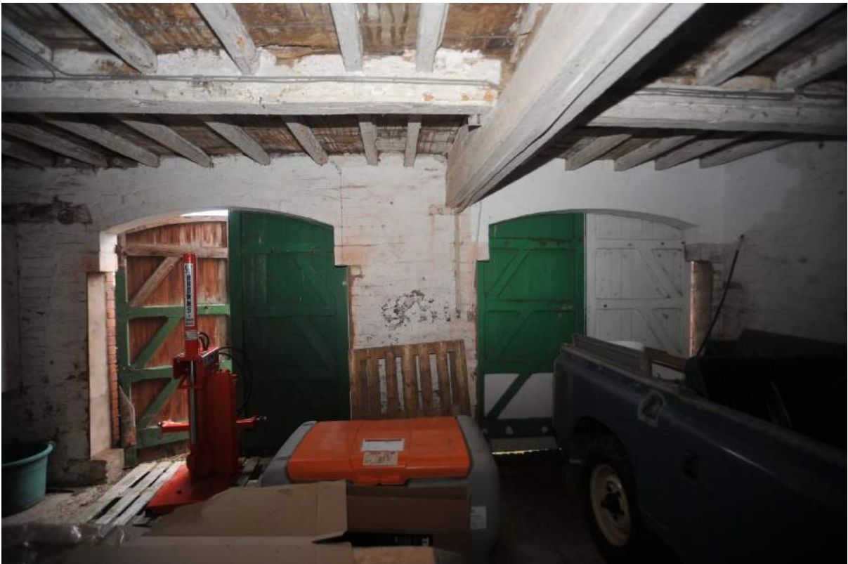
Pl.32: Interior of the eastern end of the West Range, the former coach house, looking north.
