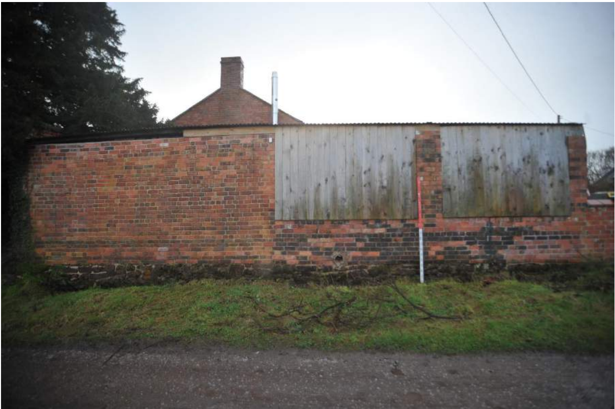
Pl.38: North side of outbuilding to north of East Range, with East Range gable beyond.
