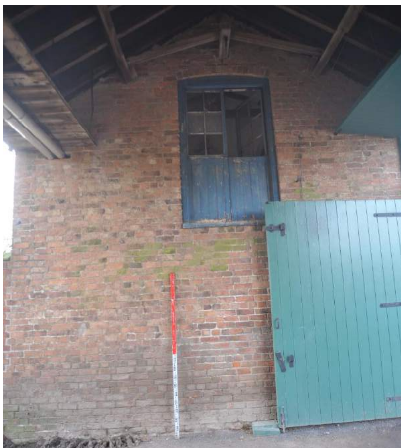
Pl.16: South side of the drift-way through the East Range.
