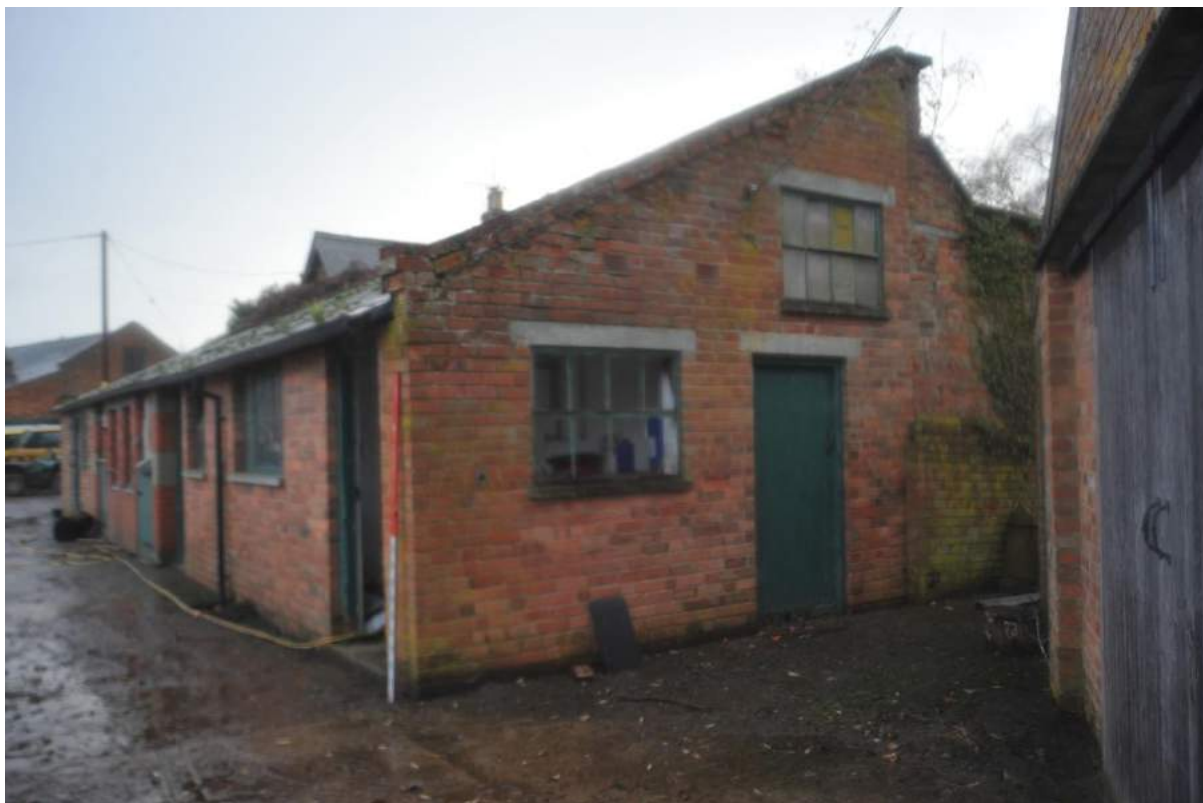
Pl.43: Modern stables at west end of complex, viewed from the west.
