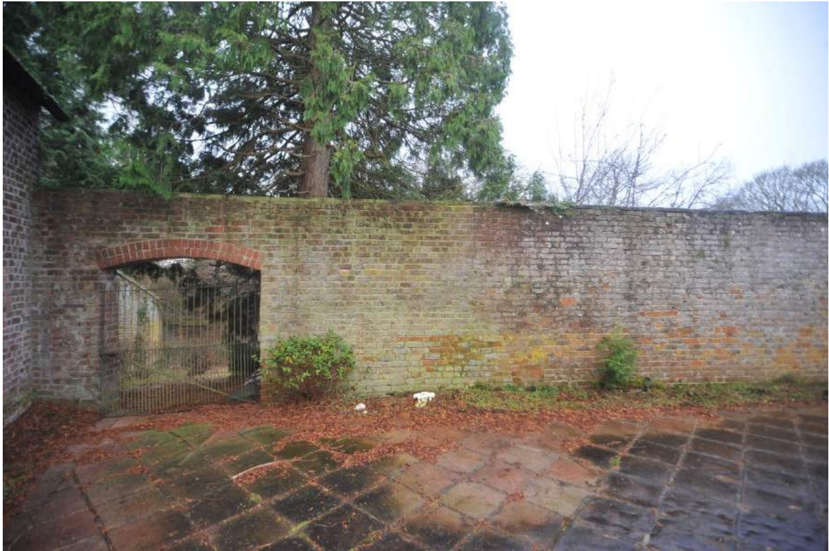
Pl.48: Part of the north side of the north garden wall south of the outbuildings complex.
