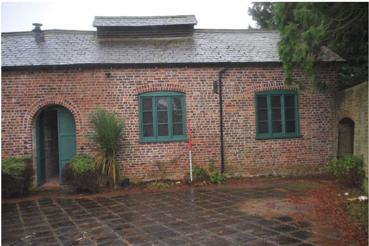
Pl.14: Southern end of the west elevation of the East Range.
