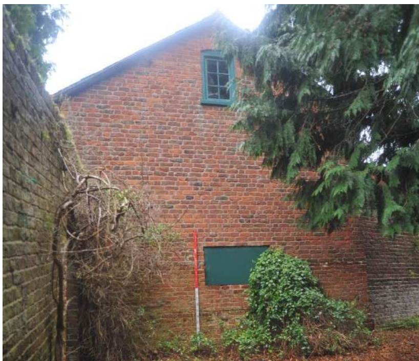
Pl.15: South gable of the East Range.
