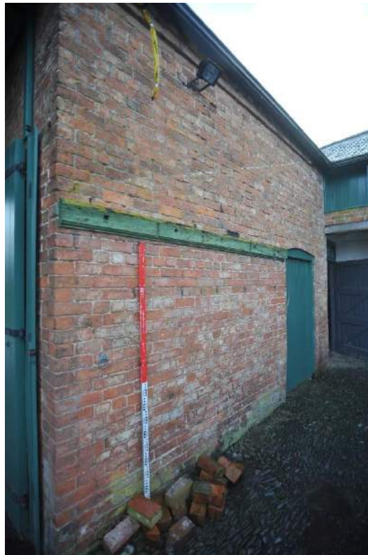
Pl.12: West elevation of the East Range to south of the drift-way.
