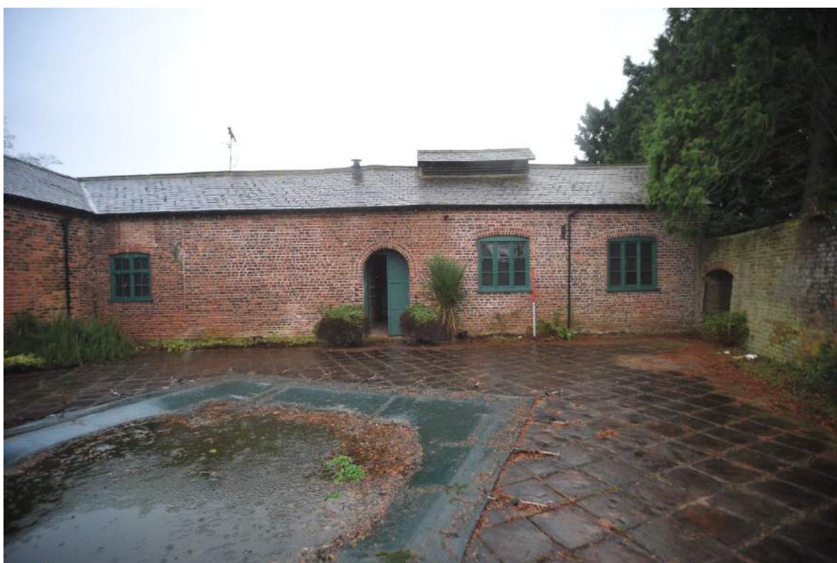
Pl.4: The southern end of the west elevation of the East Range.
