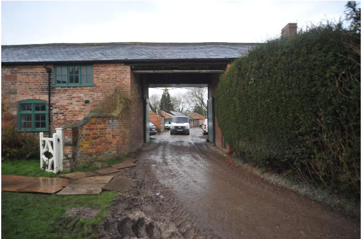
Pl.9: The east side of the drift-way through the East Range.
