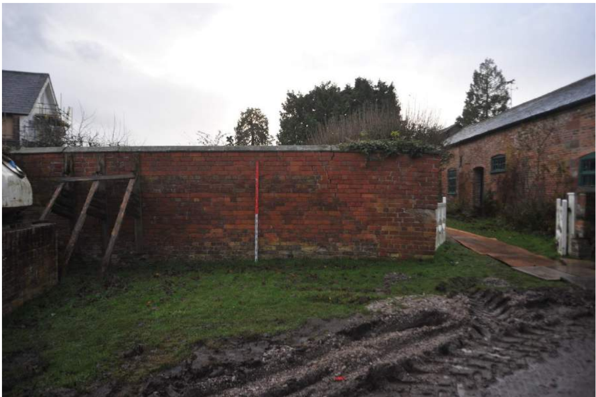
Pl.55: North side of the wall and gateway to the rear of the main house, East Range to right.
