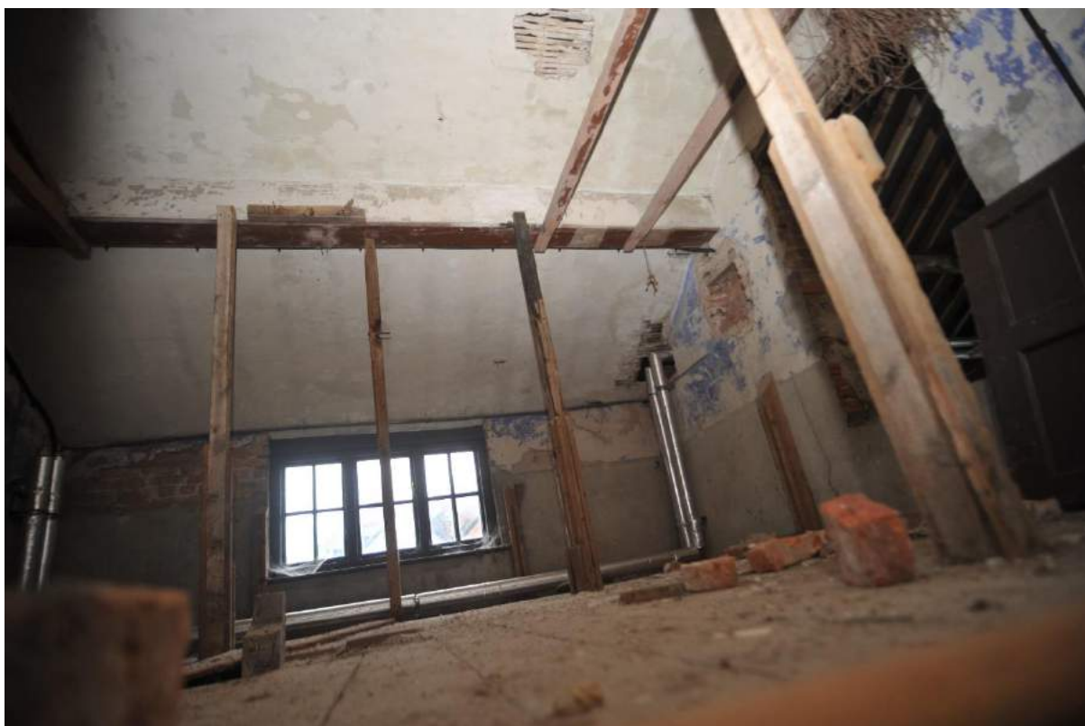
Pl.27: Part of loft above the northern half of the East Range.
