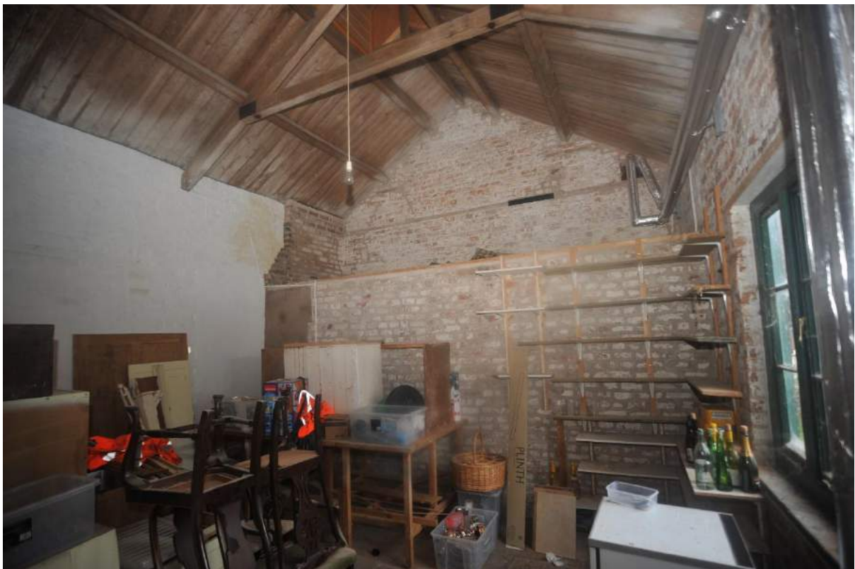
Pl.22: Penultimate southern ground-floor space in the stable of the East Range, looking north.
