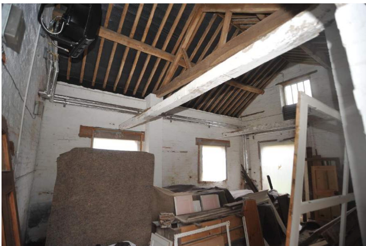
Pl.34: West end of the West Range, looking south-west.
