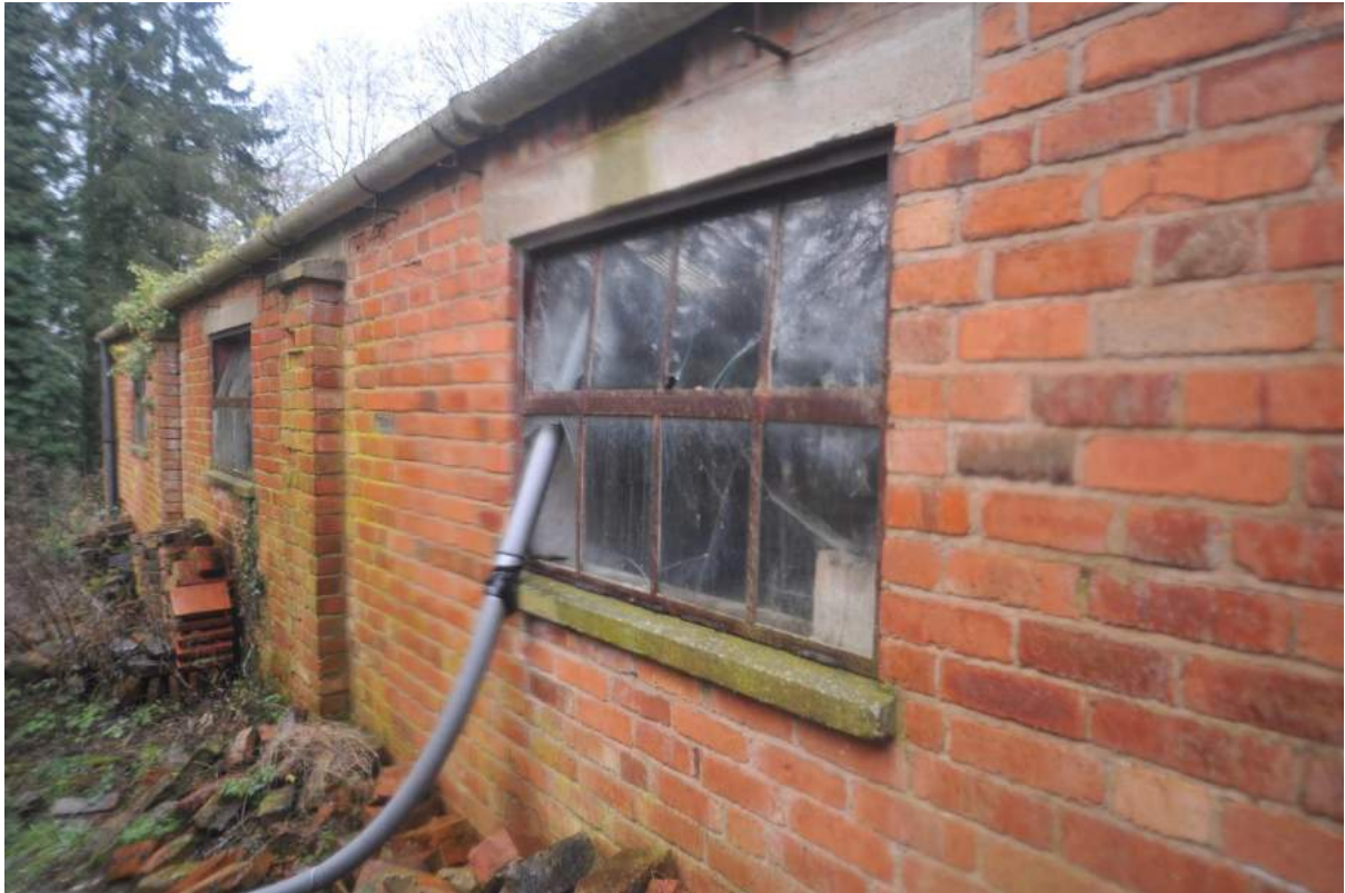
Pl.46: South elevation of the mid-20 th century byre.
