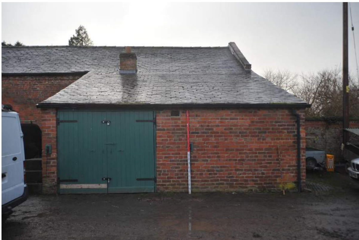
Pl.29: West end of the north side of the West Range, including lean-to extension.
