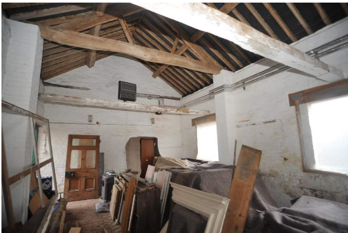
Pl.35: West end of the West Range, looking east.
