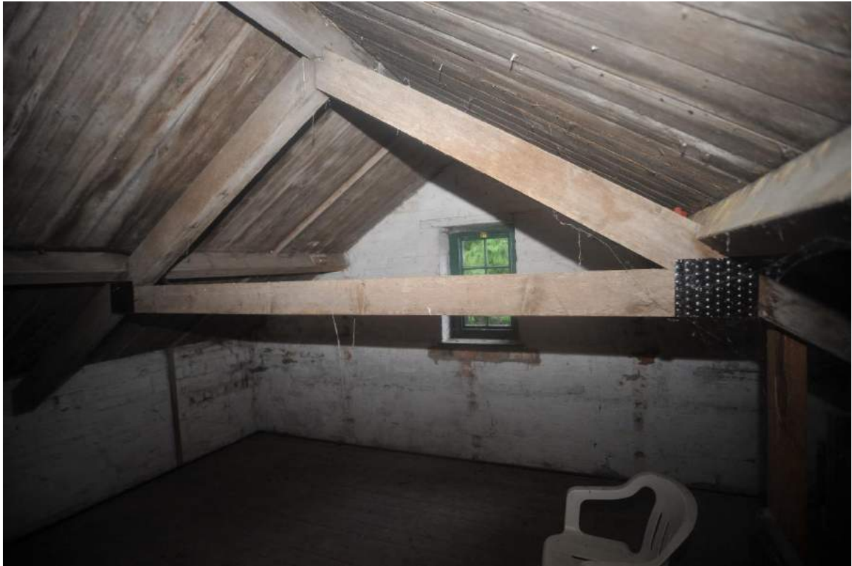
Pl.25: Southern loft space in the Barn Range, looking south.
