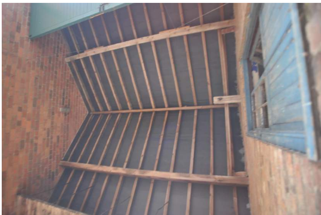
Pl.18: Roof of the drift-way through the East Range.
