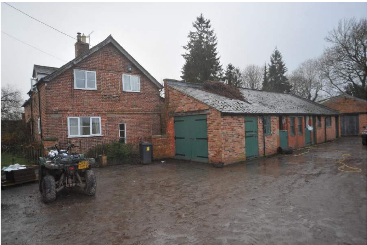
Pl.40: North side of Cottage converted from coach house, with Stables to the right.
