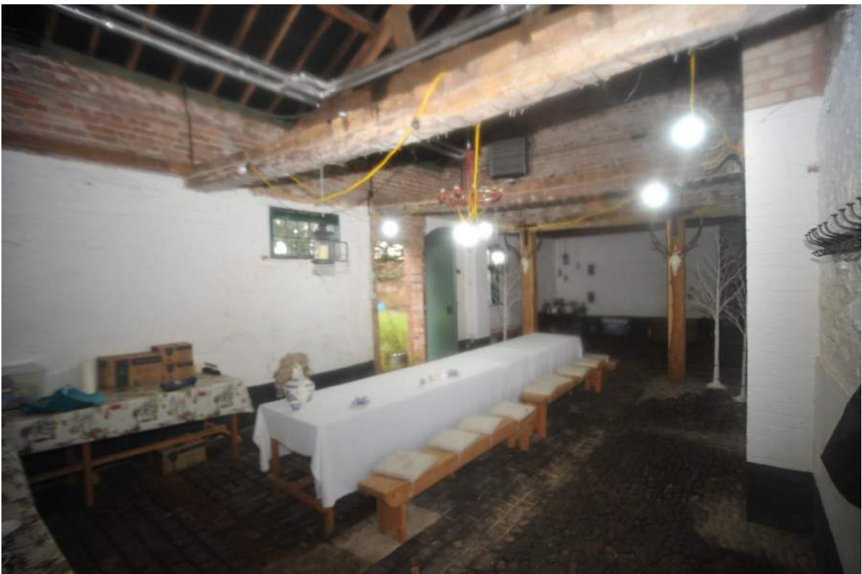
Pl.20: Barn section of the East Range, looking south-east.
