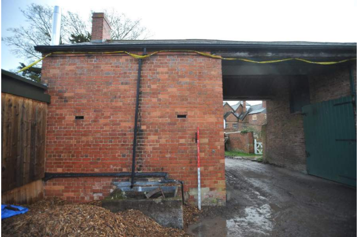
Pl.11: The northern end of the west elevation of the East Range.
