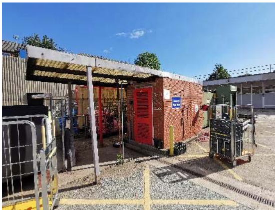
Photo 3. Exterior of building B2.
