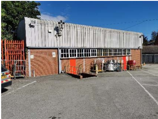
Photo 1. Exterior of building B1 with external security lighting.
