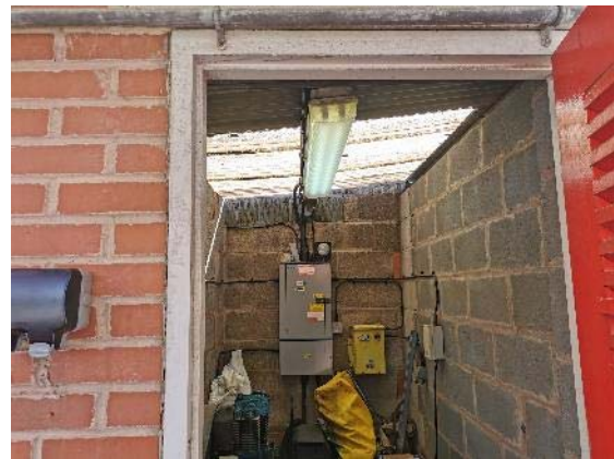
Photo 4. Interior of B2 with skylight.
