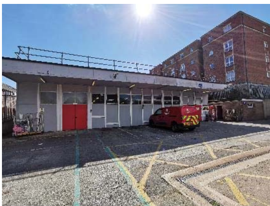
Photo 5. Frontage of building B3.
