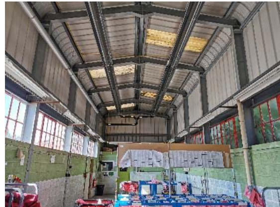
Photo 2. Interior of building B1 with steel frame roof structure, windows and sky lights.
