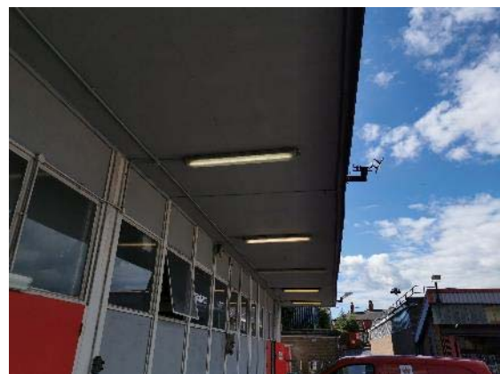
Photo 6. Underneath of overhang of building B3.
