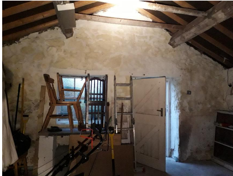
PHOTO 4.3 SOUTHERN GABLE END
