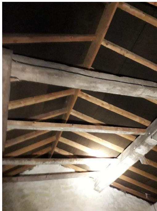
PHOTO 4.4. EXPOSED ROOF STRUCTURE
