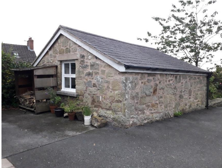
PHOTO 4.1 NORTH WESTERN CORNER OF THE BUILDING
