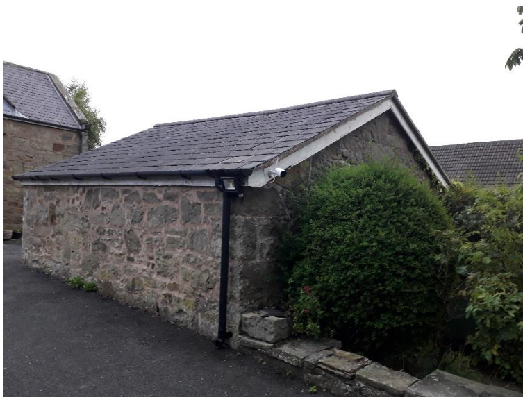
PHOTO 4.2 SOUTH WESTERN CORNER OF THE BUILDING
