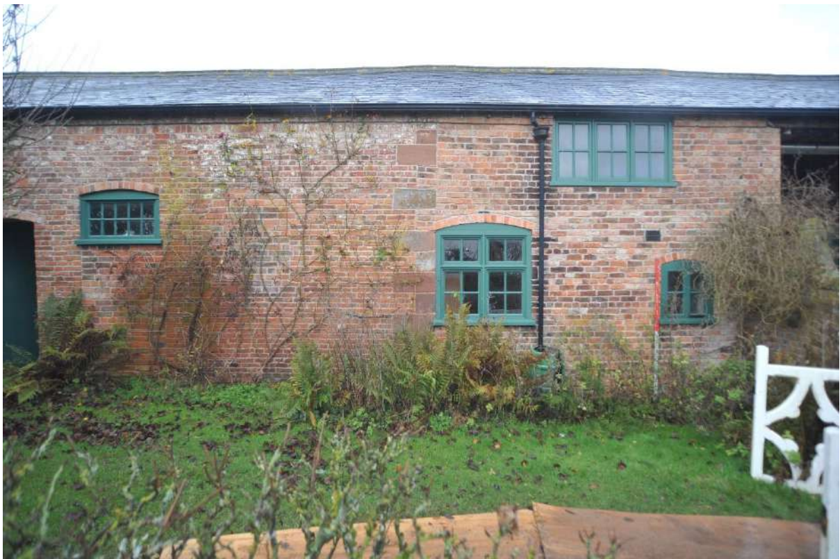
Pl.8: Part of the central section of the east elevation of the East Range.
