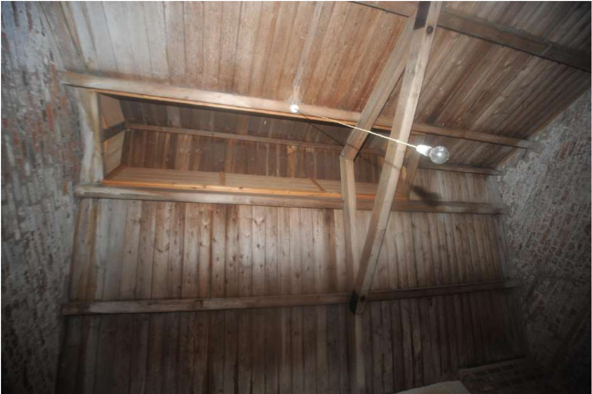
Pl.23: Roof and louvre over the penultimate southern room in the stable of the East Range.
