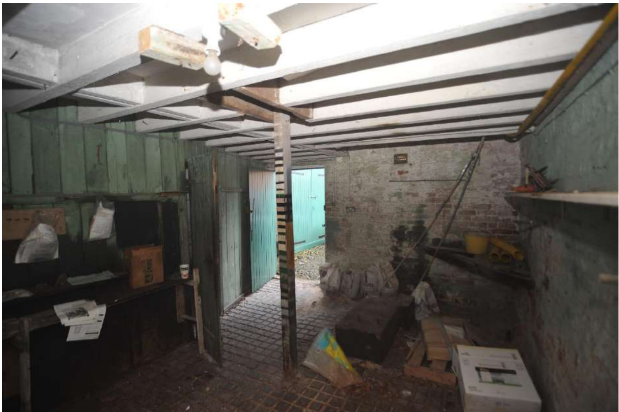
Pl.26: Stable south of drift-way in the East Range.
