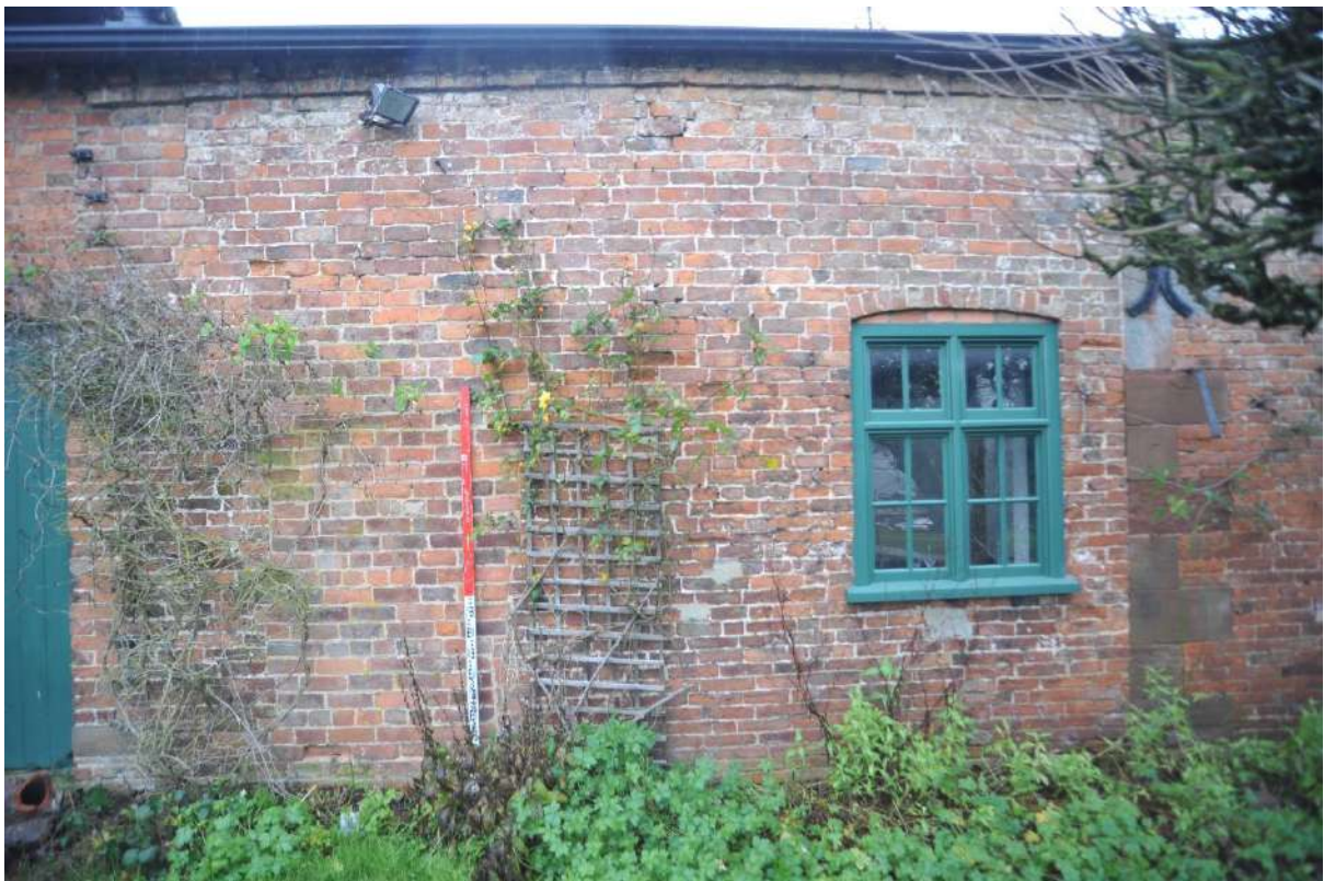
Pl.6: Part of the southern part of the east elevation of the East Range.
