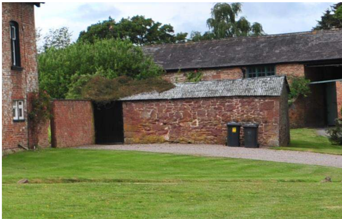
Pl.52: Stone outbuilding to north of house from the east.
