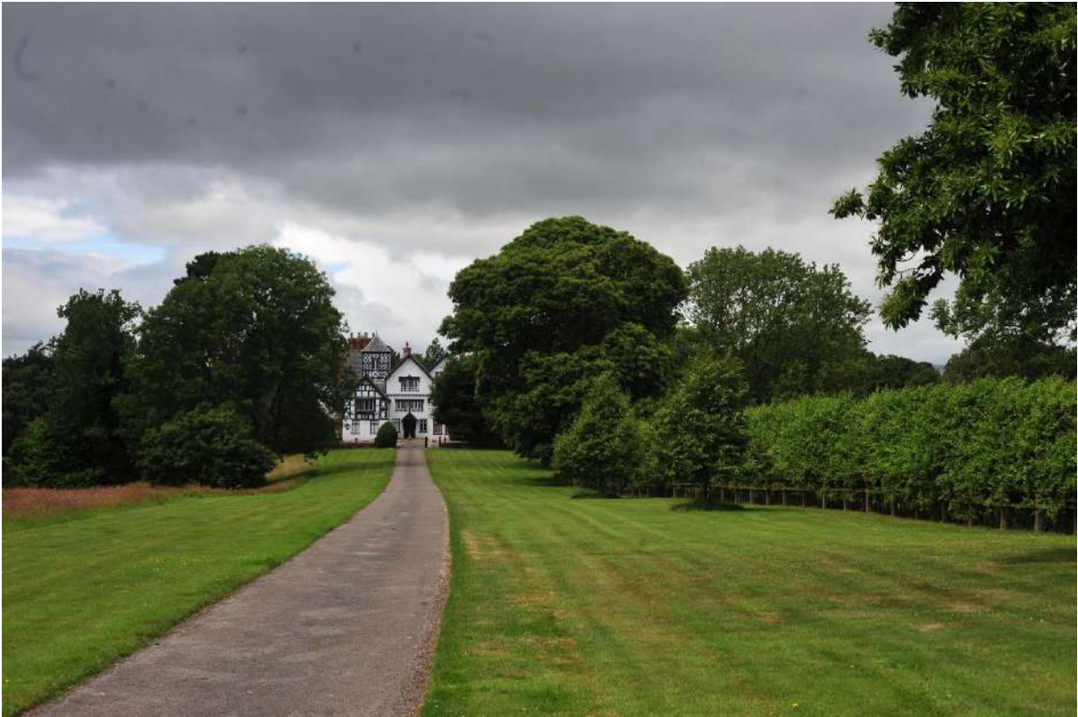
Pl.1: The east, or entrance front, of Knolton Hall viewed from the drive.
