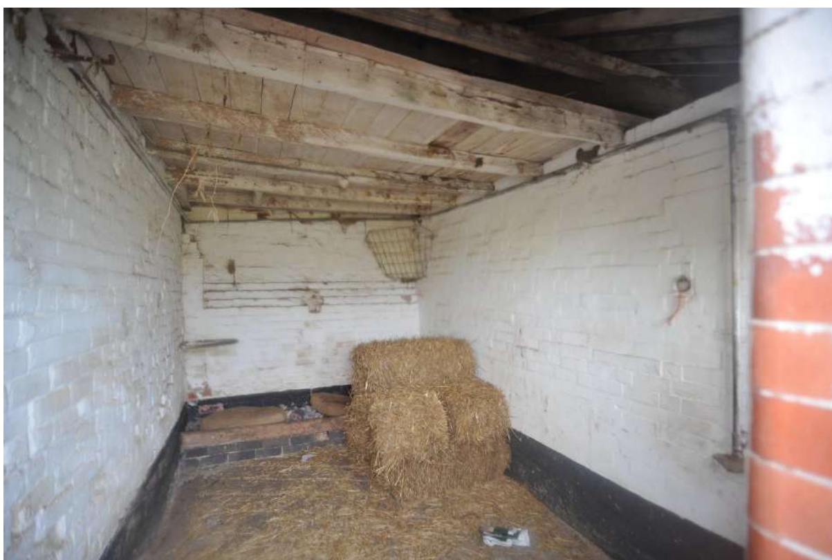
Pl.44: Typical interior stall in the modern stables.
