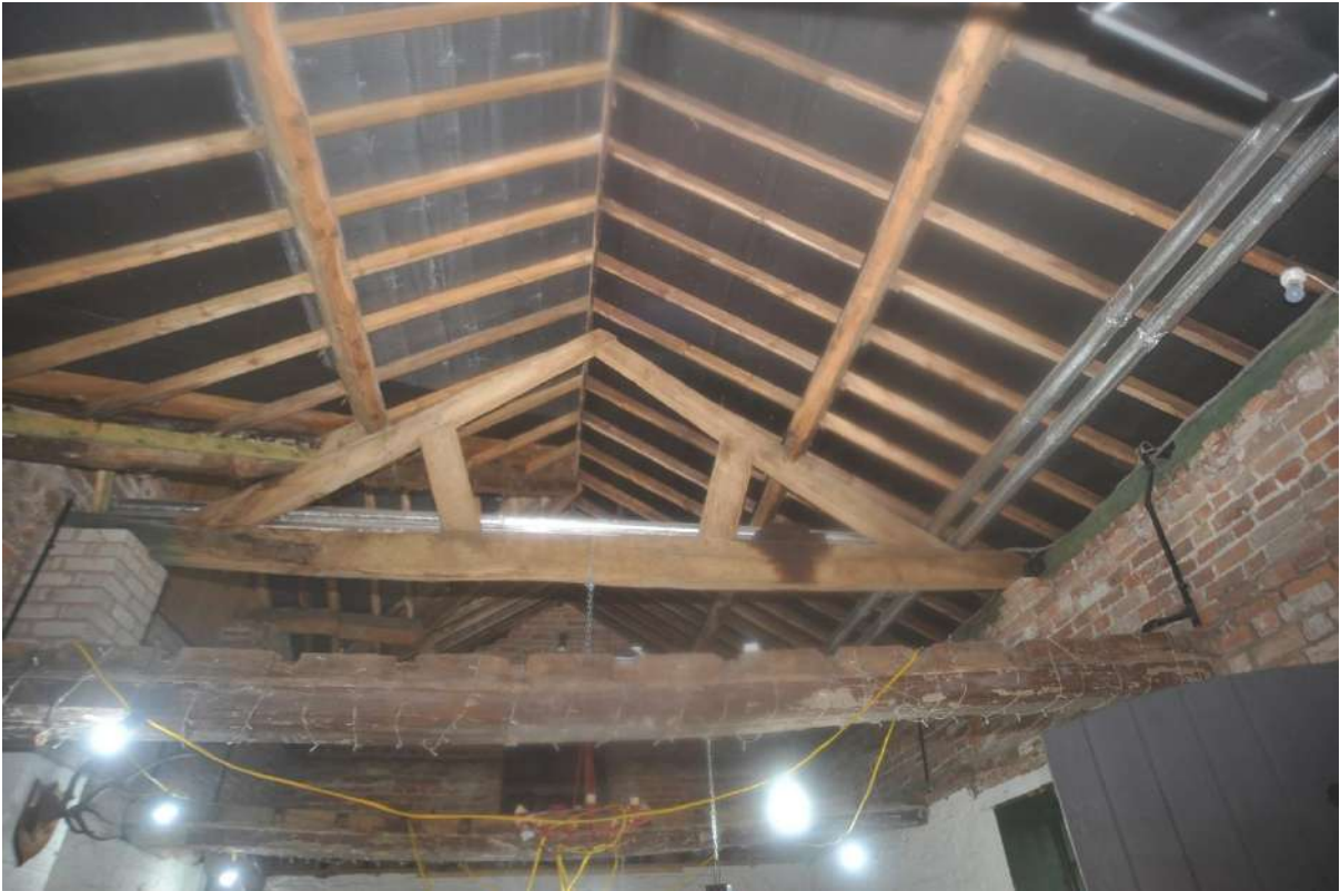
Pl.19: Roof structure over the barn section in the East Range.
