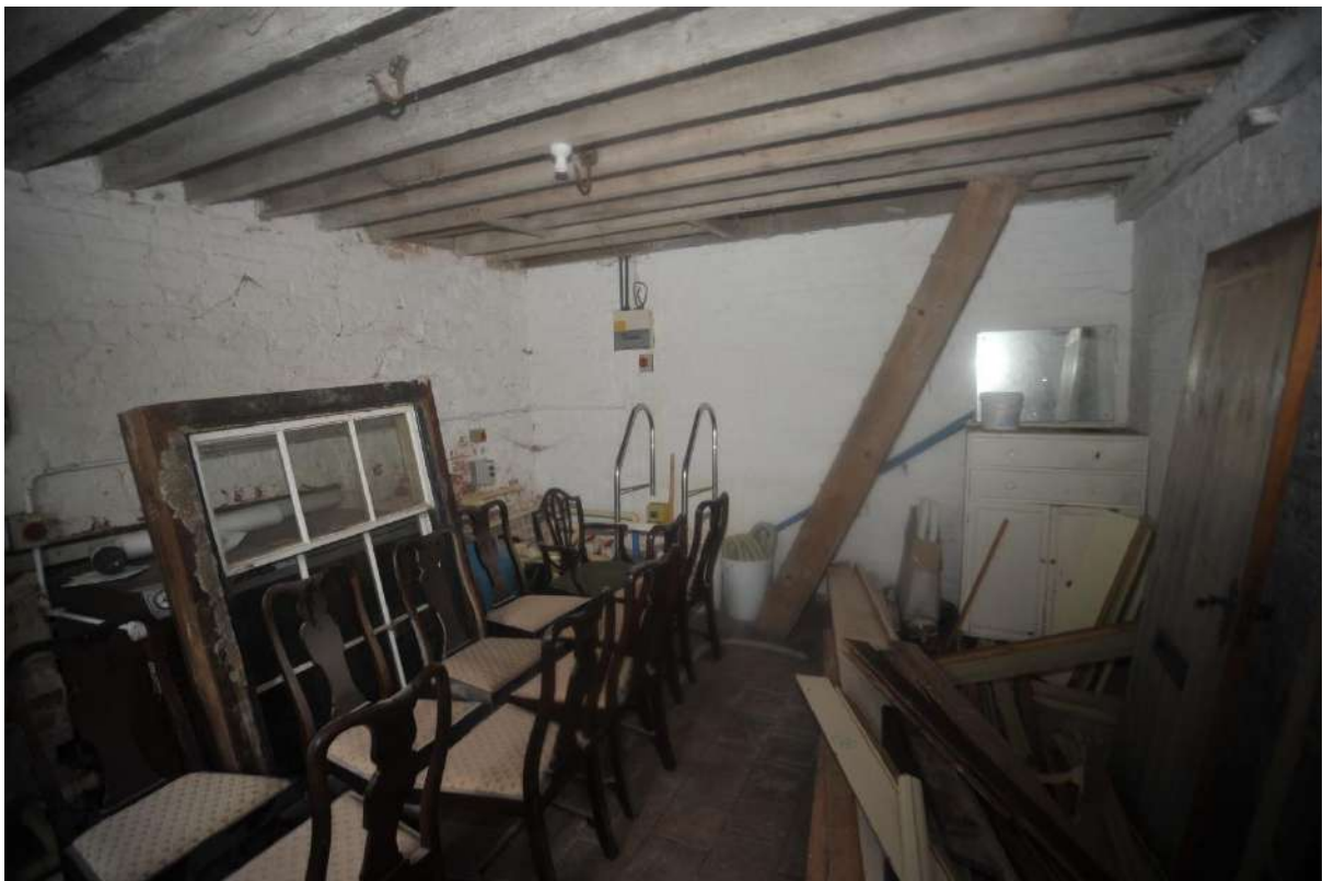
Pl.24: Southernmost ground-floor room in the Barn Range, looking west.
