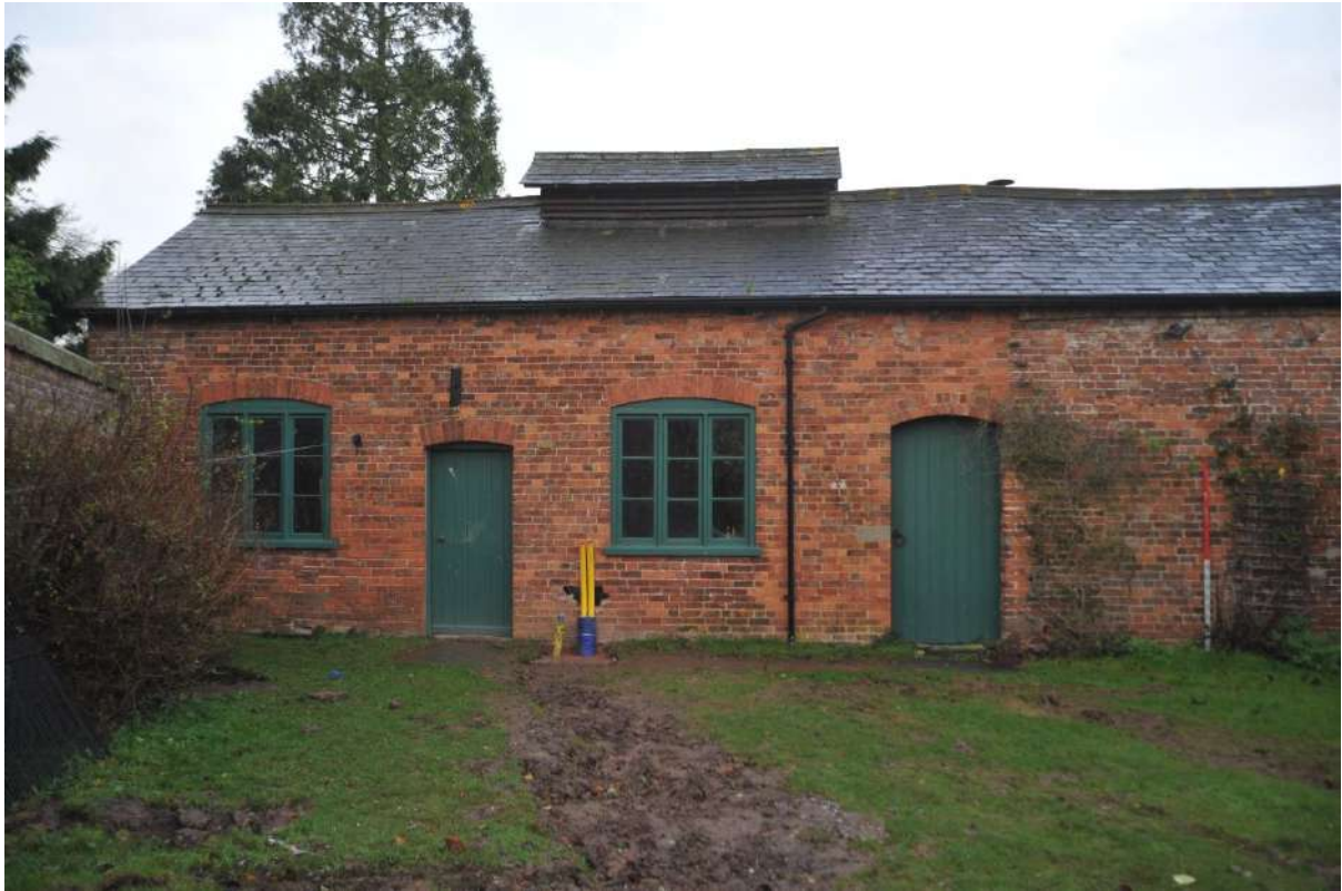
Pl.5: Southern end of the east elevation of the East Range.
