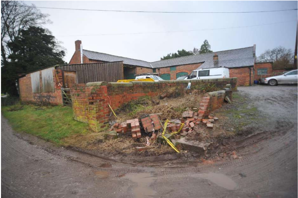
Pl.50: General view of the complex from the north-west with walled yard in foreground.
