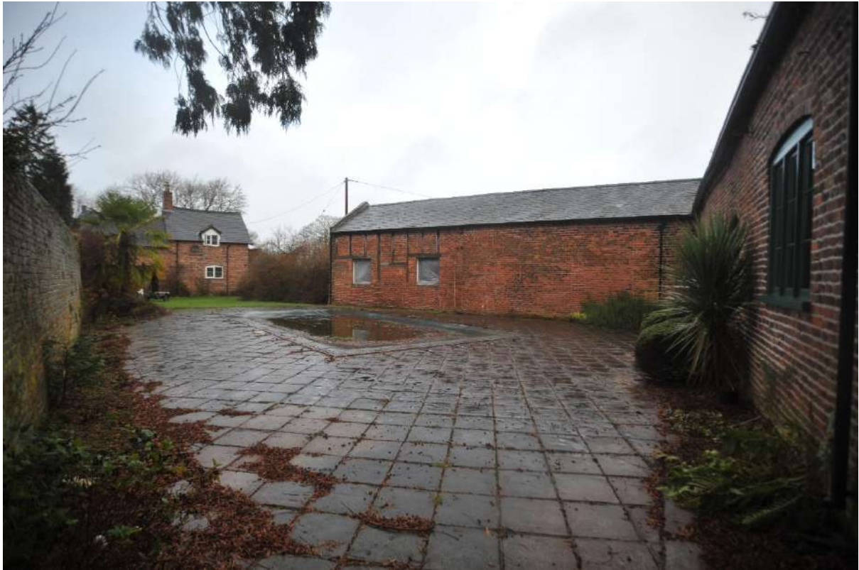
Pl.39: View of south yard area westwards towards converted cottage in background, left.
