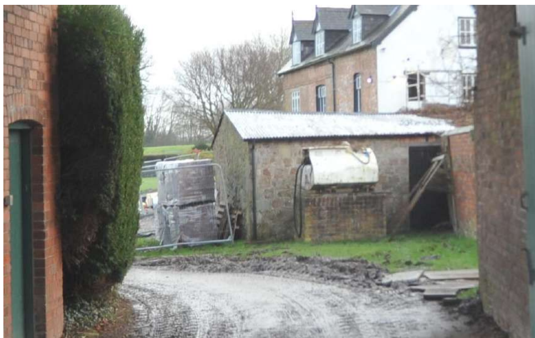
Pl.53: Stone outbuilding from the west, viewed through the driftway.
