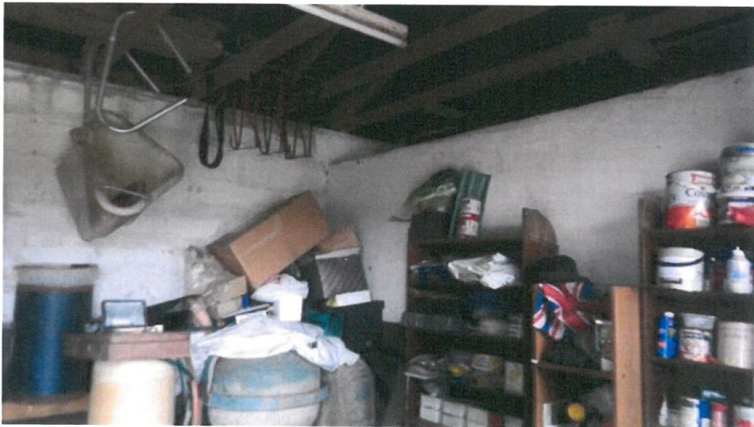
Plate 9 The stables are currently used as a general storage area; all surfaces were check for bat droppings.
