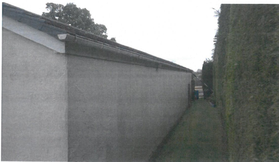
Plate 3. The building is well sealed with no gaps or crawl areas. The fascia is sealed to the rendering.
