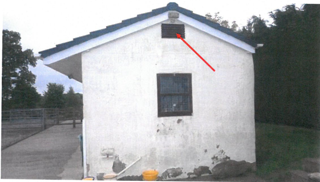
Plate 2. The building offers little roosting potential for bats. All the brickwork is well pointed and sealed and the roof is in good condition. The vents appeared to be the only access point, however on close inspection they were sealed internally.
