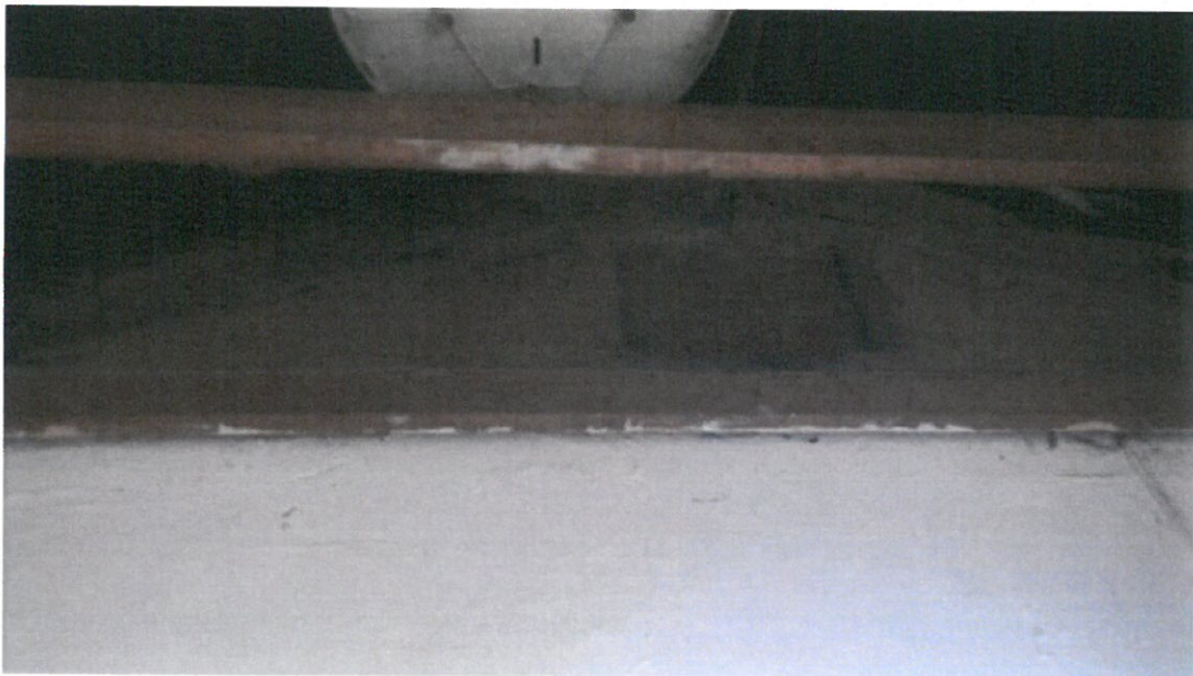
Plate 7 The external vents were sealed via a board which prevents any access to the building.
