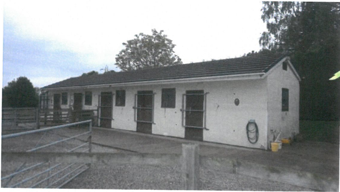
Plate 1. The building is a stable building set on hard standing.
