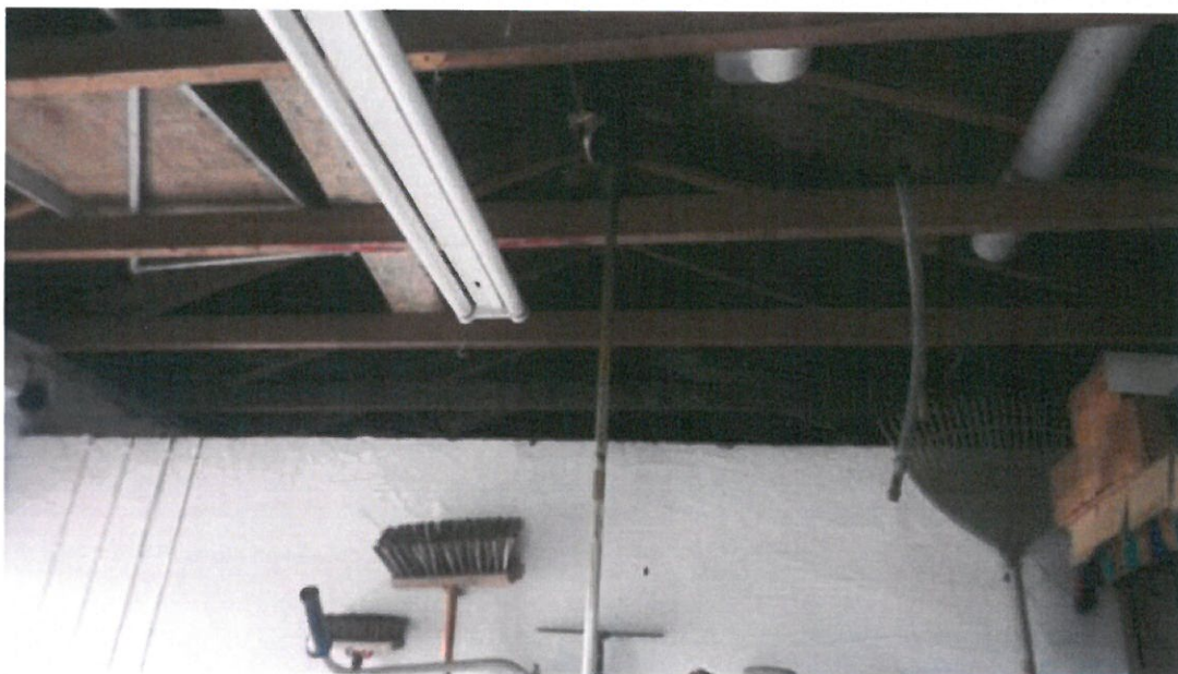
Plate 5. No loft space occurs within the building, the internal area is wide open, however the area was extensively searched for signs of bat presence – none were found. The roof is lined with a bitumen membrane, which seems in good overall condition.
