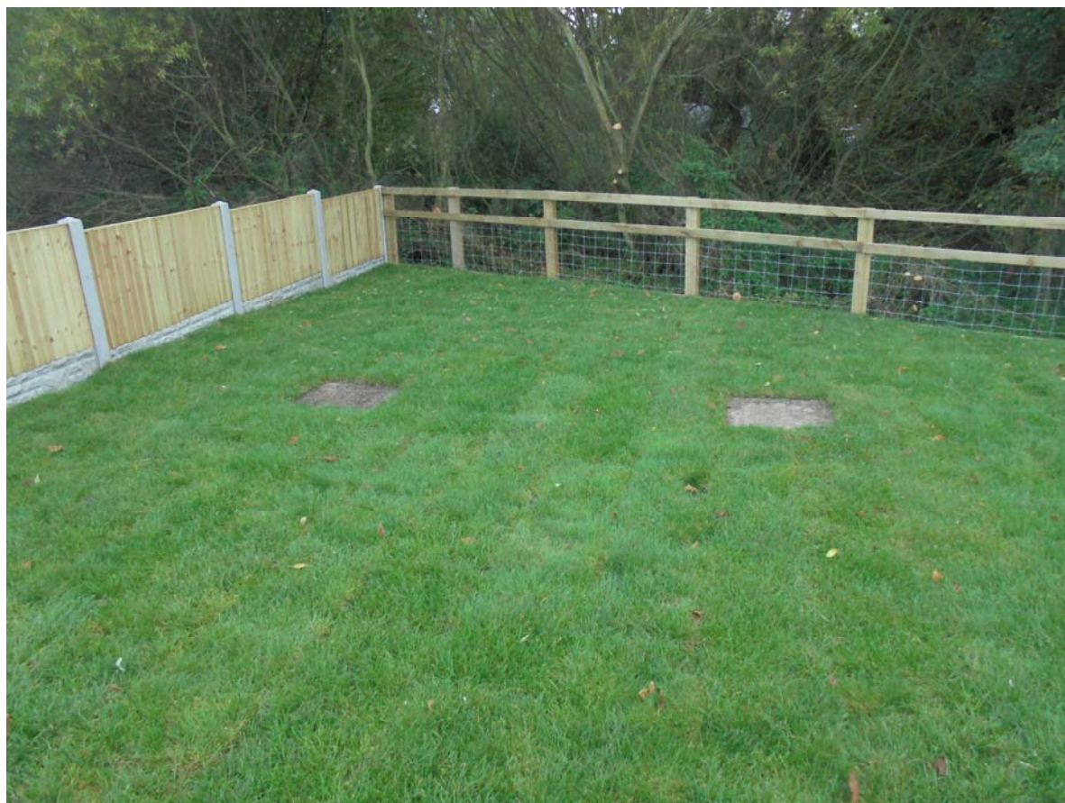
Photo 3 – Downstream manhole covers located within rear garden of 5 White House Mews. Removable fence panels providing access. Hydrobrake flow control chamber on left.
