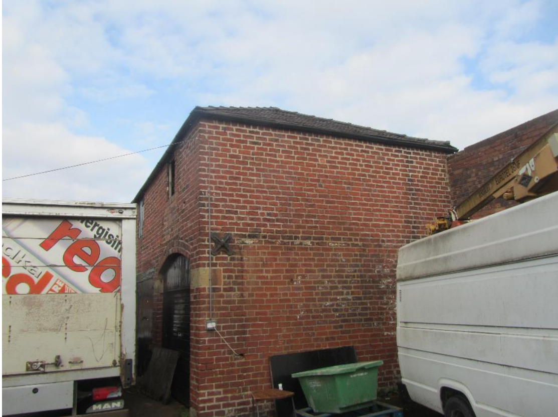
Image 3.25 Western elevation of B3
