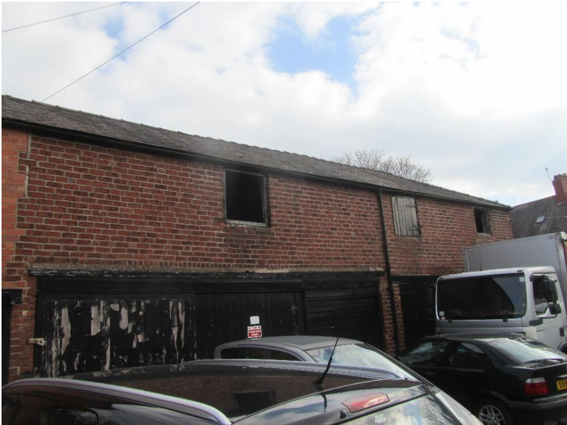
Image 3.26 Northern elevation of B3
