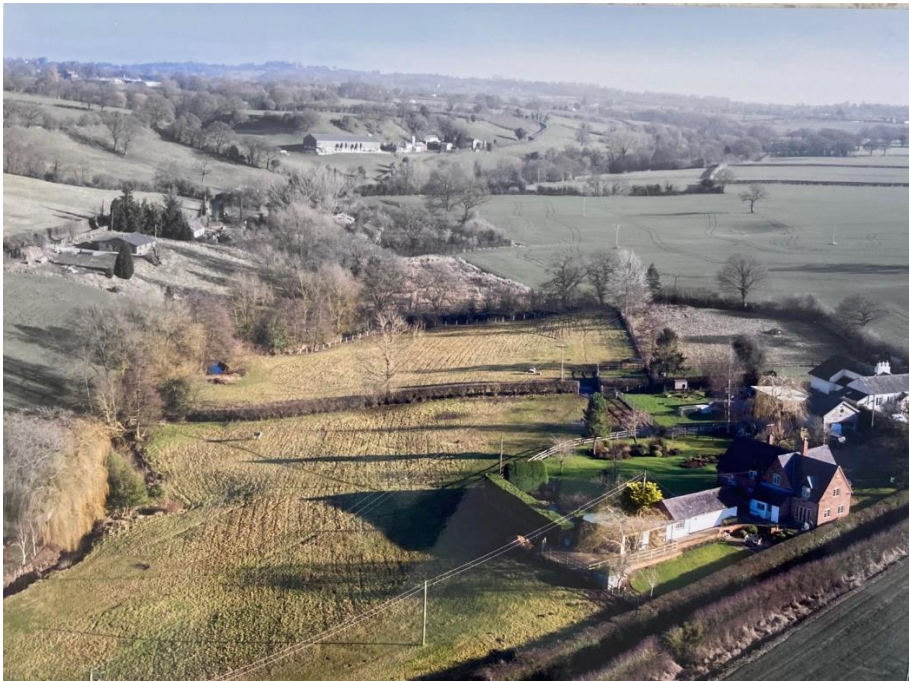
Fig 1. Aerial view of the site with the boundary stream to the left of shot.
