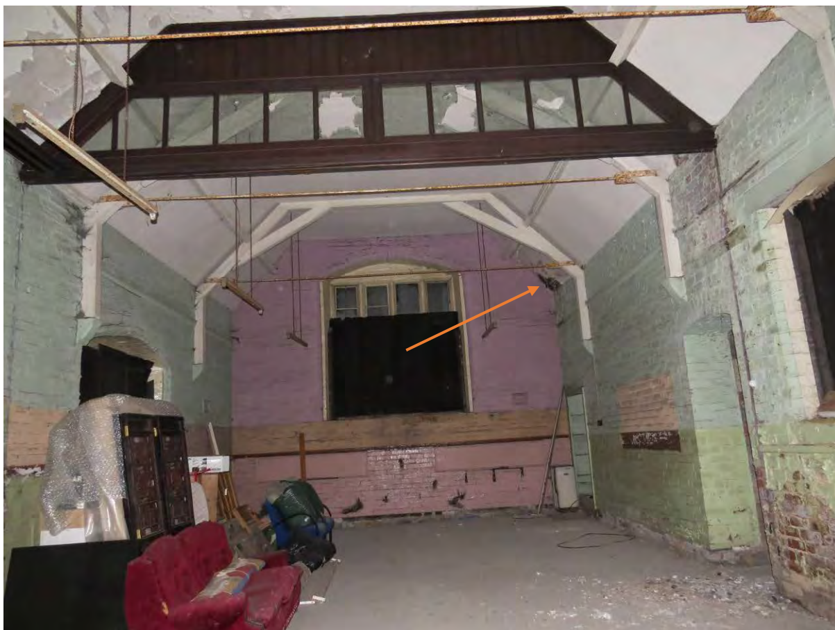
12. The interior of the part of the southern section where a lesser horseshoe bat was roosting during the scoping survey.
