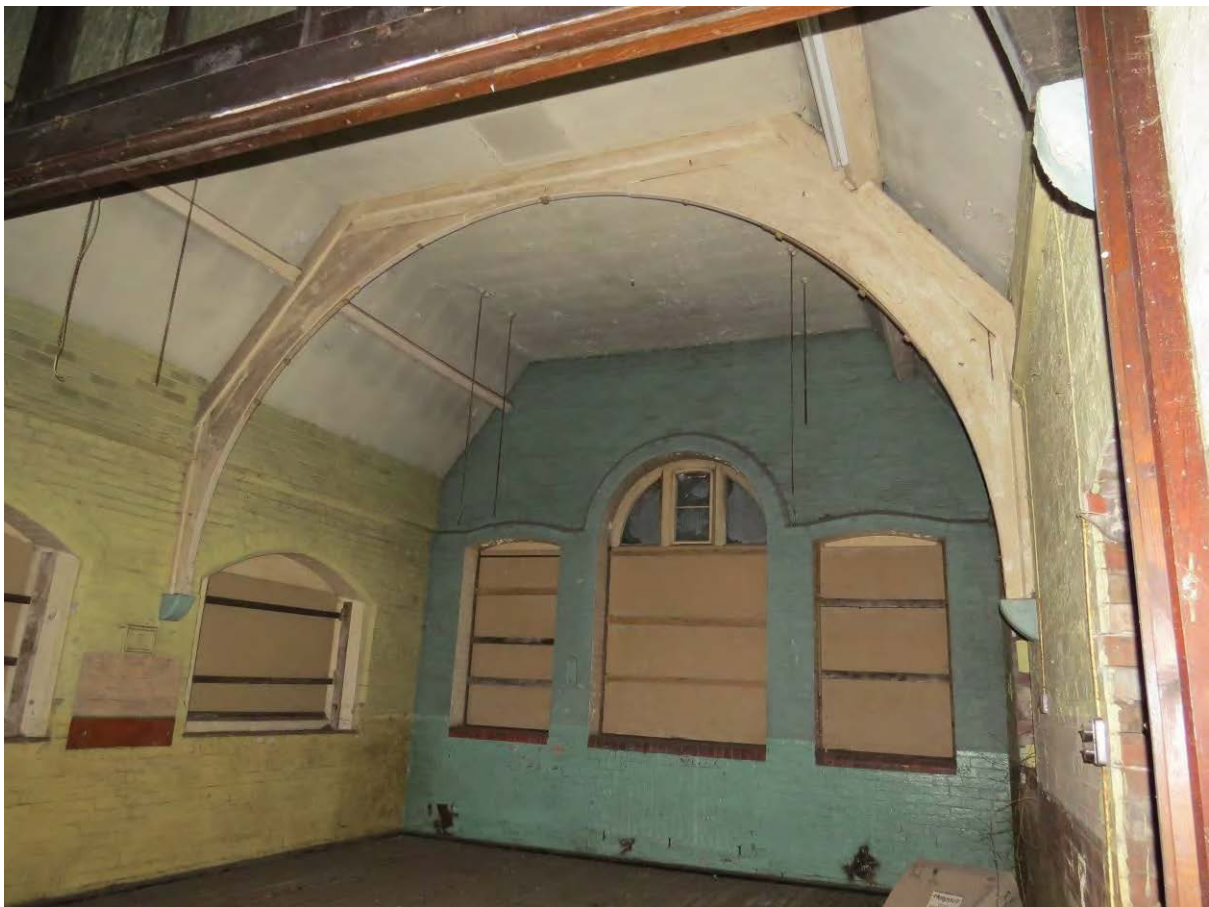
8. The interior of the northern section of the building.
