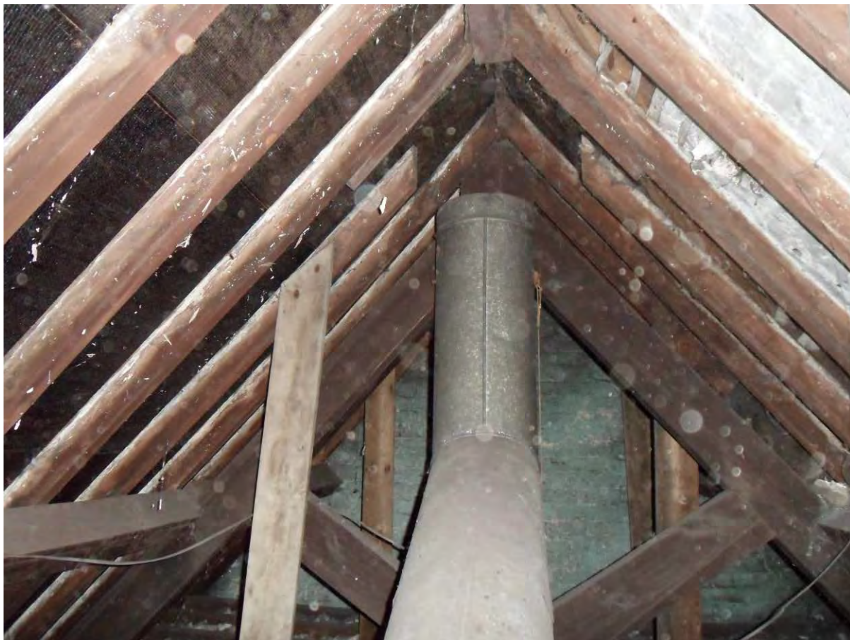
17. Part of the southern roof space.
