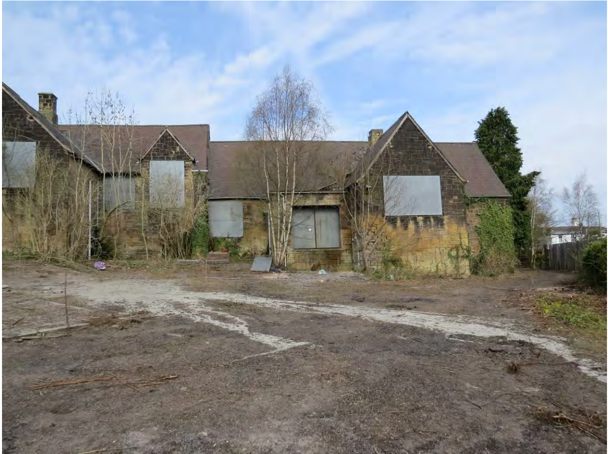
3. Looking west towards the rear of the school building.
