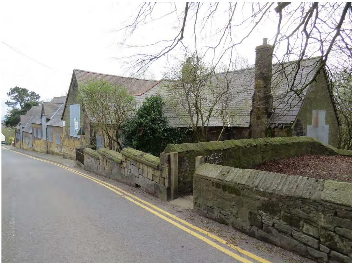
2. Looking north along High Street with the southern gable end of the school on the right.
