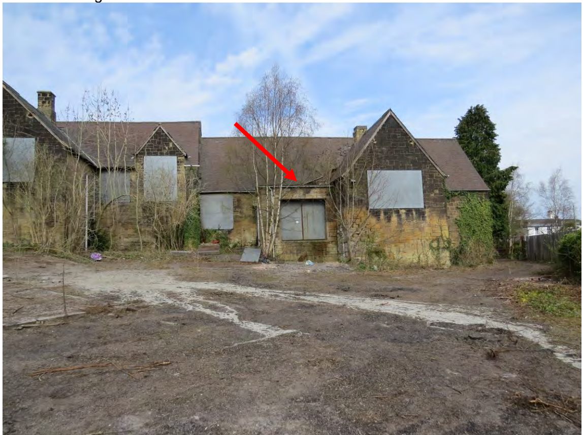
C.5b – Looking towards the roost entrance (a perished flat roof) from ground level.
