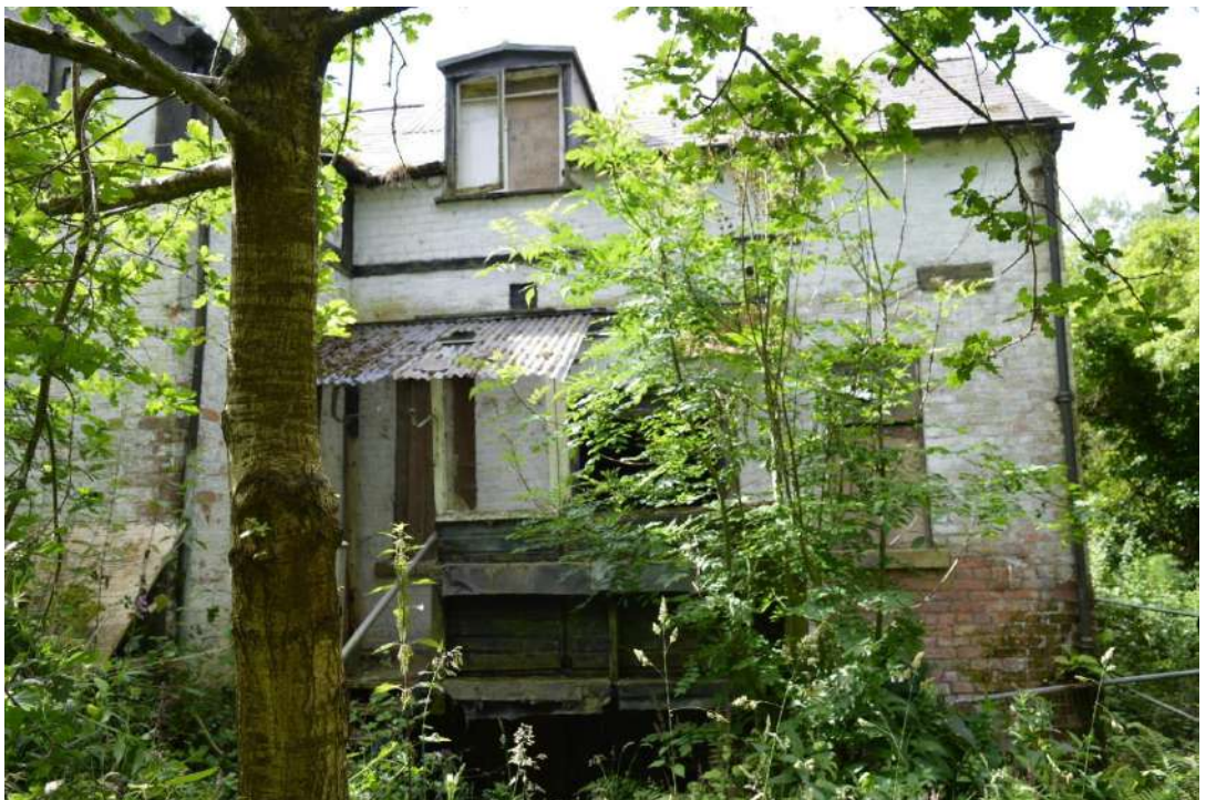
Fig. 8. Northern elevation of the mill. CPAT photo 4661-0030.
