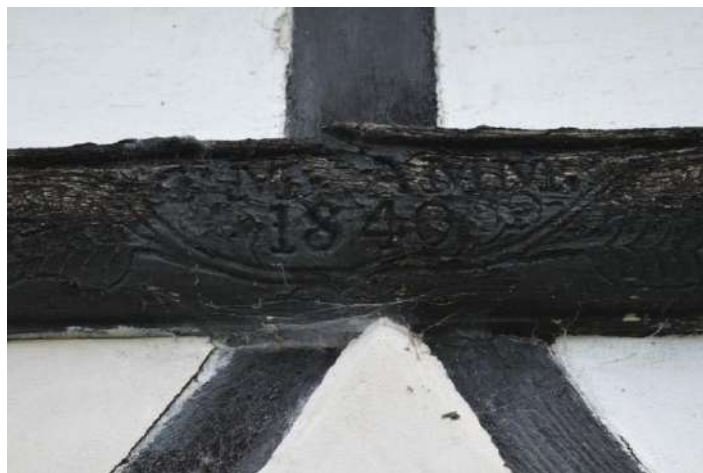
Fig. 6. Date carved on the southern elevation of the mill house. CPAT photo 4661-0021.
