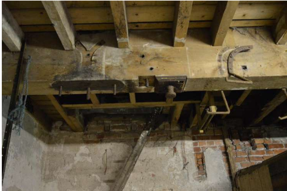
Fig. 10. Fixings to the mill beams, viewed from the east. CPAT photo 4661-0059.
