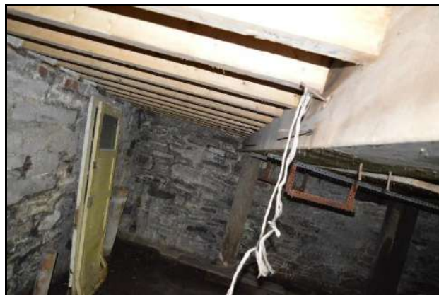
Fig. 11. View of the mill cellar from the north. Note the large timber upright and the yellow doorway thorough the eastern elevation into the mill house. CPAT photo 4661-0048-49.
