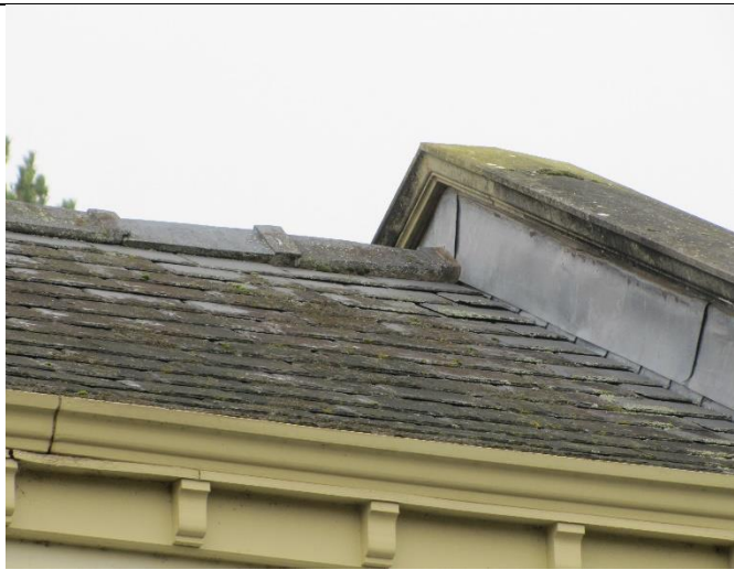
Detail showing well-bedded slates and ridge tiles, design of eaves, gutter and parapet
