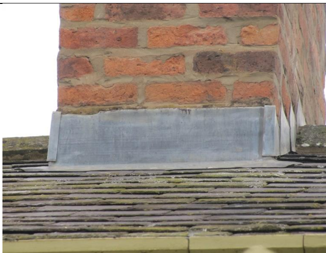
Lead flashing around chimneys
