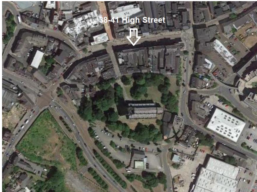
Figure 2.2 Frontage of 38-41 High Street
