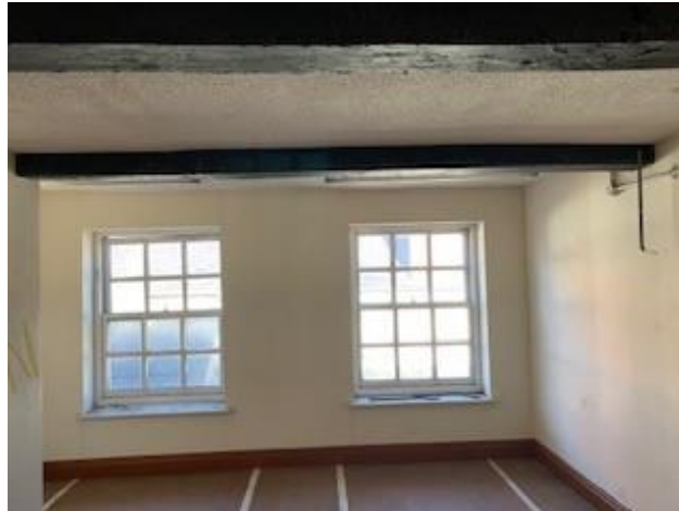
Figure 3.3 Photographs of second floor 38-41 High Street
