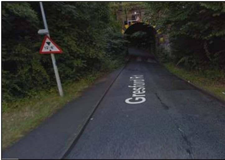
Figure 1: Low Bridge Preventing HGV Access from Gresford Road in a Southerly Direction.
