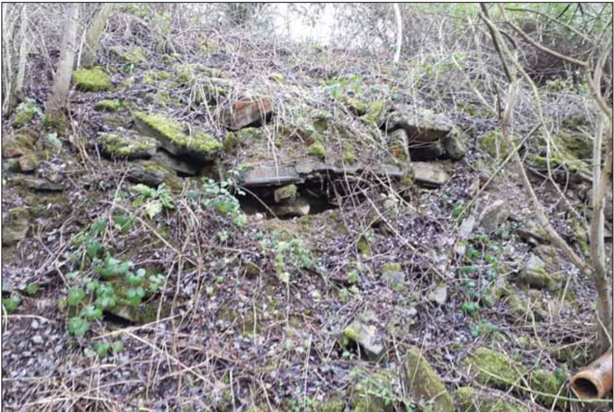
Photographs 19 & 20: Bank created from concrete demolition material originating from magazine buildings.
