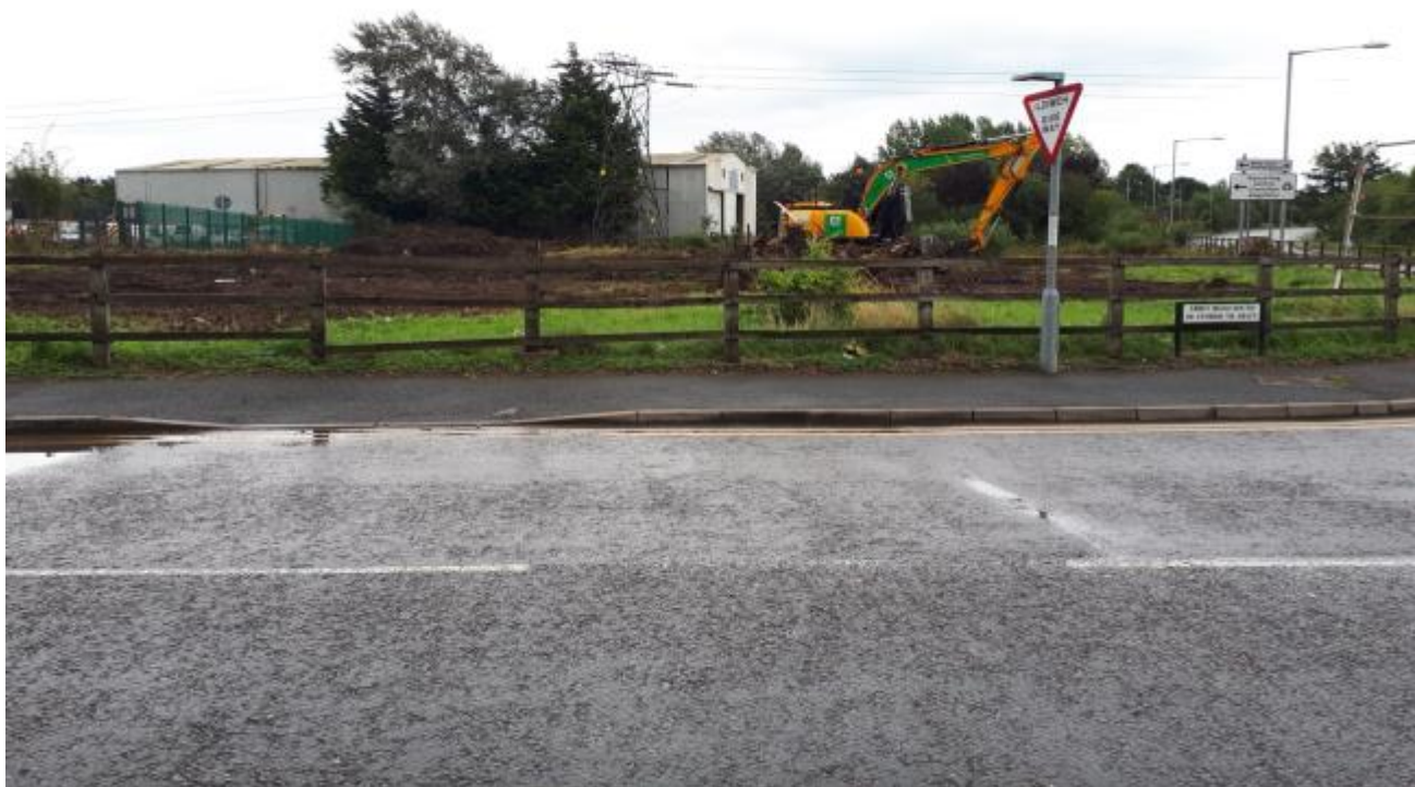
Photo 1: View East from Abbey Road South towards site. Excavator on site carrying out clearance – not operating at time of walkover.
