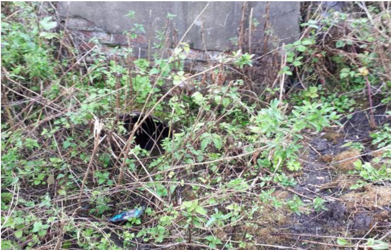
Photo 6: Drainage pipe in eastern face of concrete service cover
