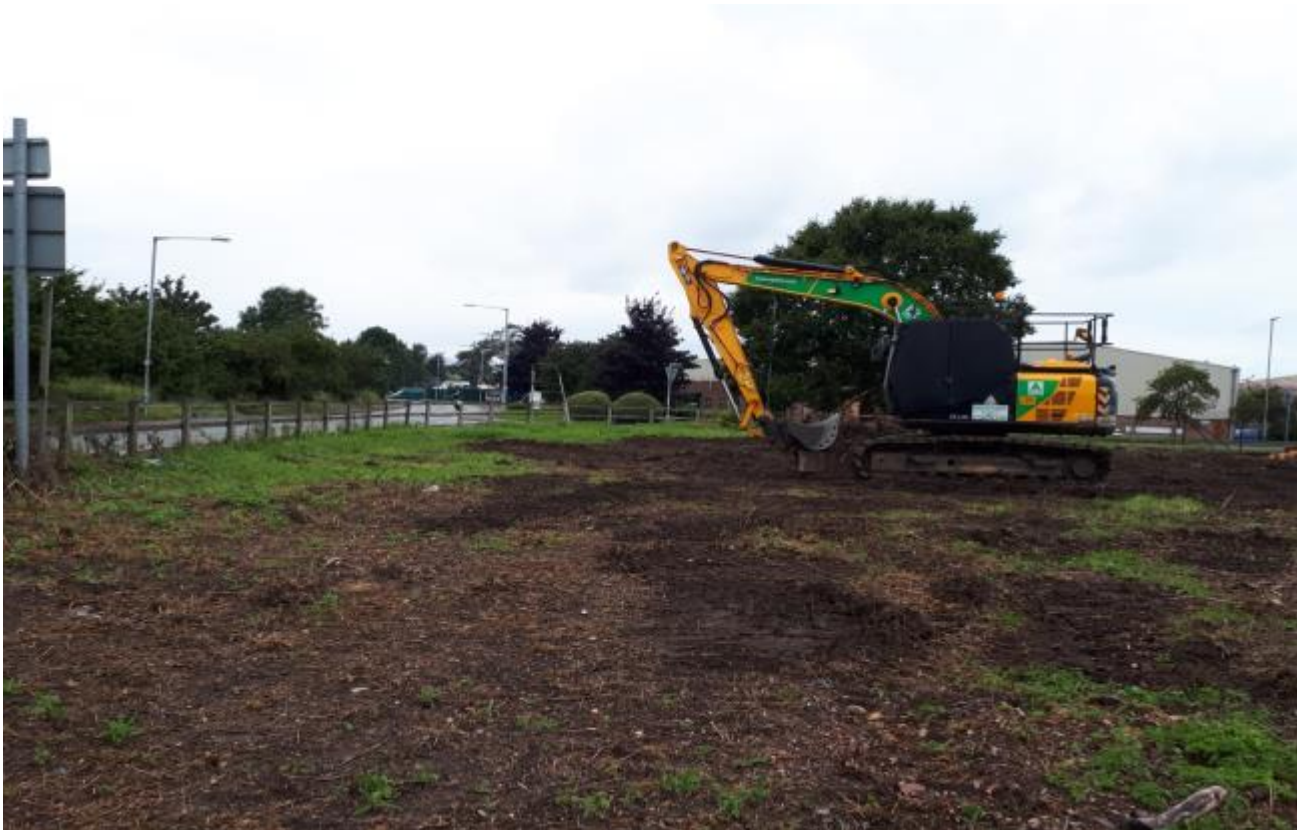
Photo 14: View West along southern site boundary
