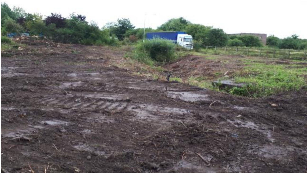
Photo 3: View East along centre of site showing concrete service cover and gully feature
