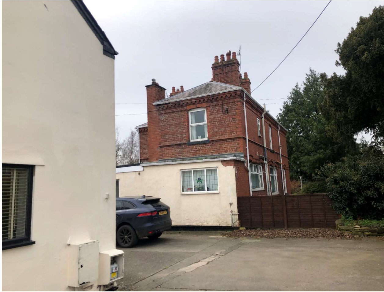
View of existing front vehicular entrance and neighbouring property Oak Lodge
