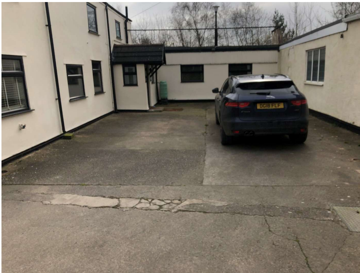
Existing front elevation, Oak Lodge to the right of the image
