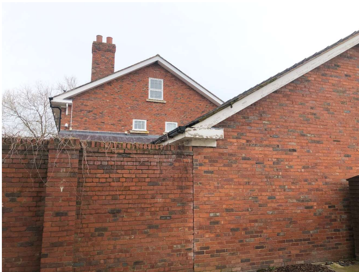
View Eastward of existing neighbouring property Drewton House and garage
