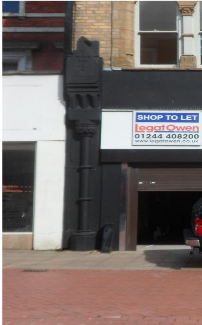
Existing black painted sandstone pilaster
