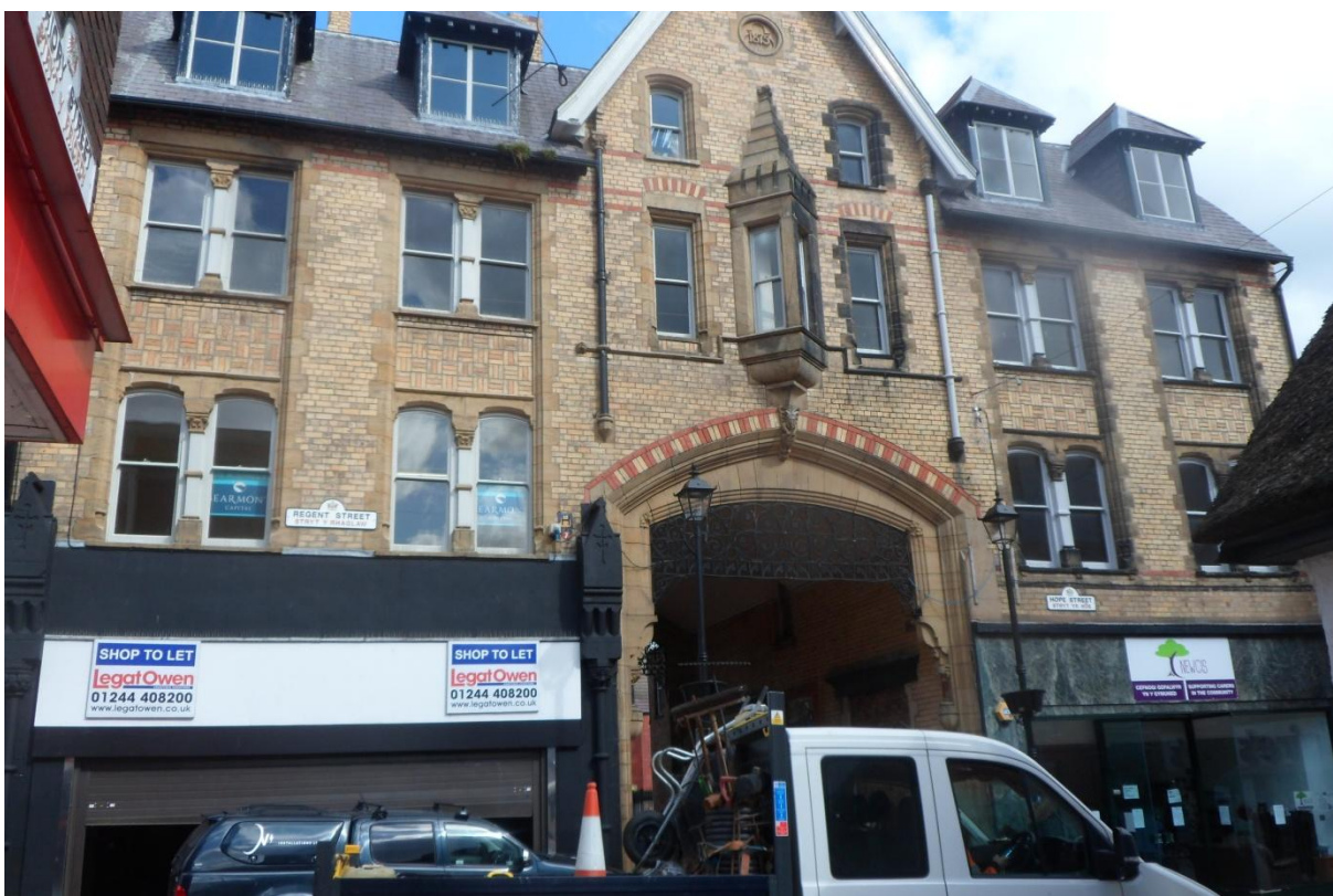
2, Regent Street to left with Archway and Neighbour
