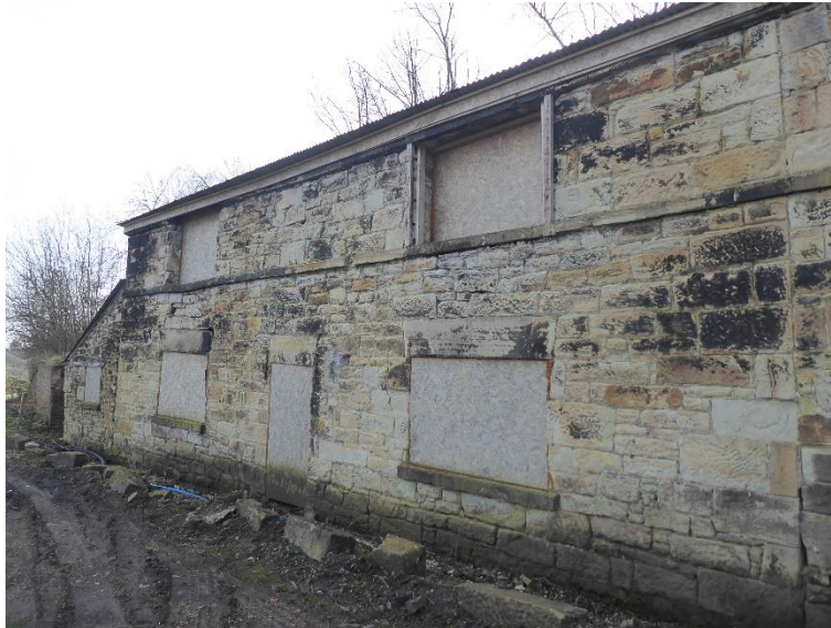
PHOTO 4.1 NORTHERN SIDE OF THE HOUSE
