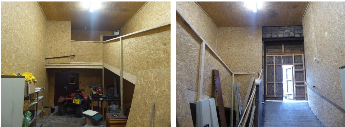
PHOTO 4.3 & 4.4. WALLS LINED WITH CHIP BOARD TO CREATE A LARGE DOUBLE STOREY HEIGHT ROOM
