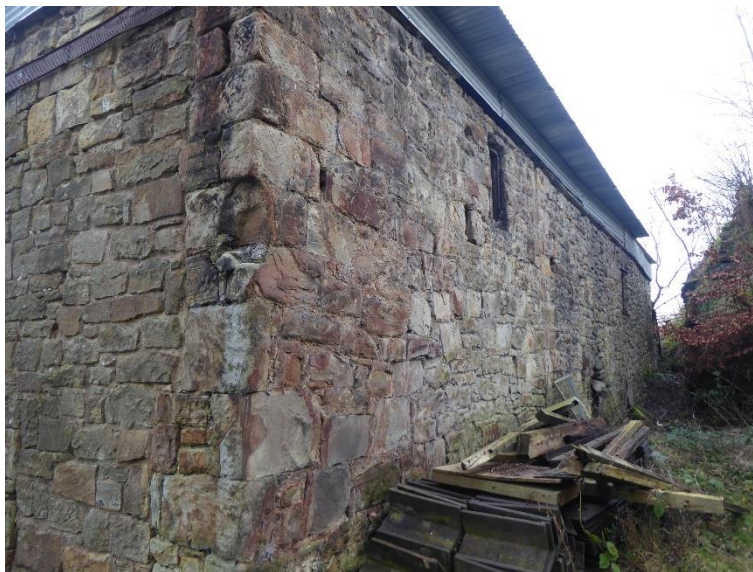
PHOTO 4.2 SOUTHERN SIDE OF THE HOUSE
