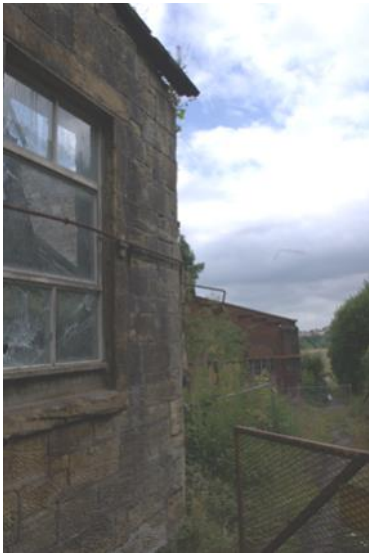
Detail of the existing metal and timber windows
