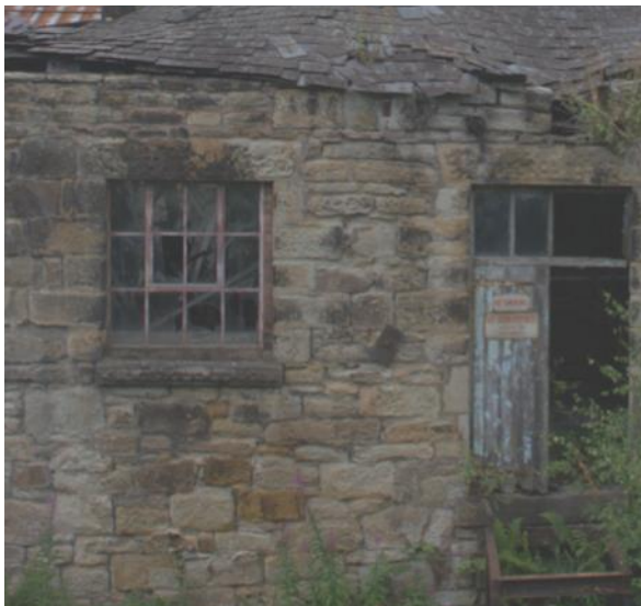
Detail of the existing metal and timber windows
