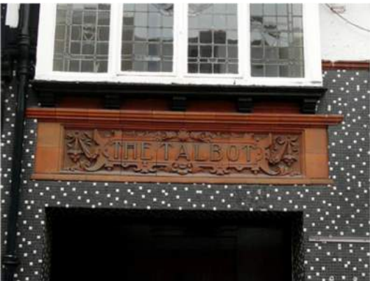
Figure 6— Terracotta Entrance sign to Talbot Inn, Queen Street.
