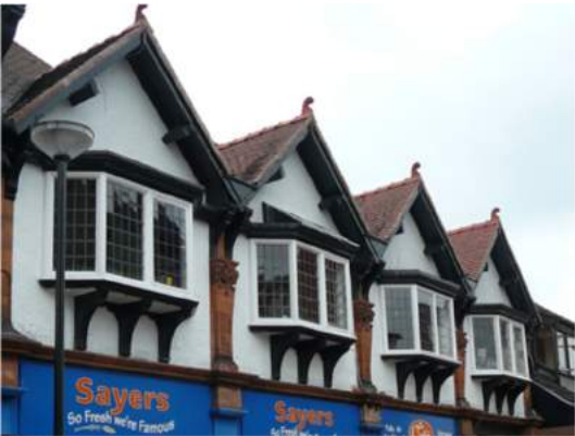
Figure 5—Gables located next to Talbot Inn, Queen Street.
